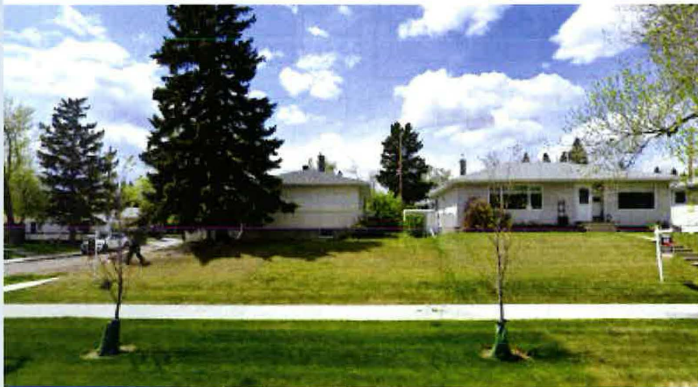
Front – 37 Street SW
