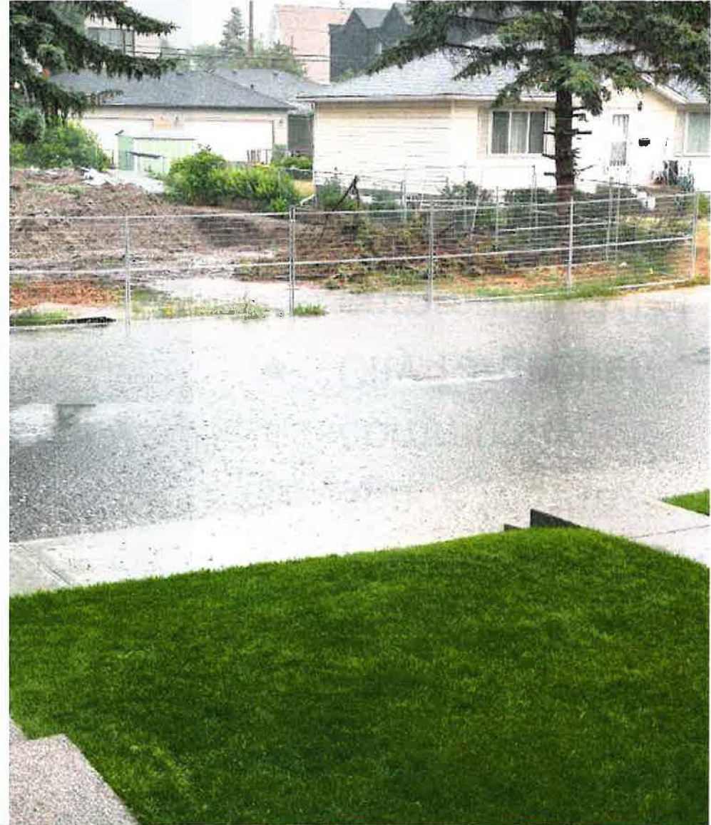
Both storm drains on 51 AVE not able to manage rainfall event - July 3, 2021
