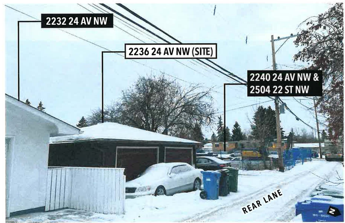
VIEW SOUTHWEST ALONG REAR LANE
