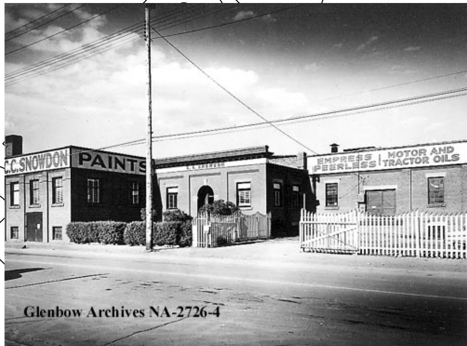
(Photo 2.5: oblique historic view of the West Façade, ca. 1950s – Glenbow Museum and Archives NA-2726-4)
