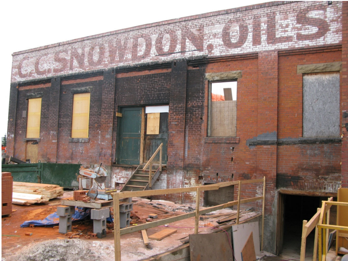
(Photo 5.2: Eastern portion of North Façade showing 1911 building section)
