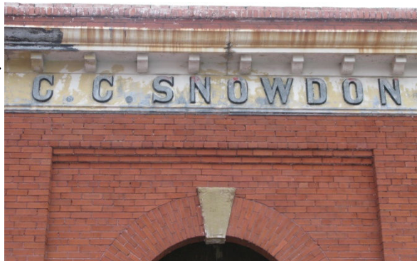
(Photo 2.9: pressed-metal roofline cornice with 'C.C. SNOWDON' lettering, 1911 building section)
