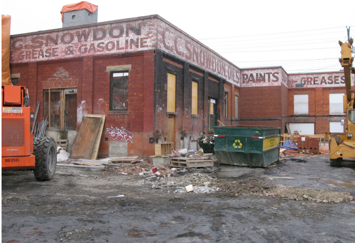
(Photo 4.2: East Façade)
