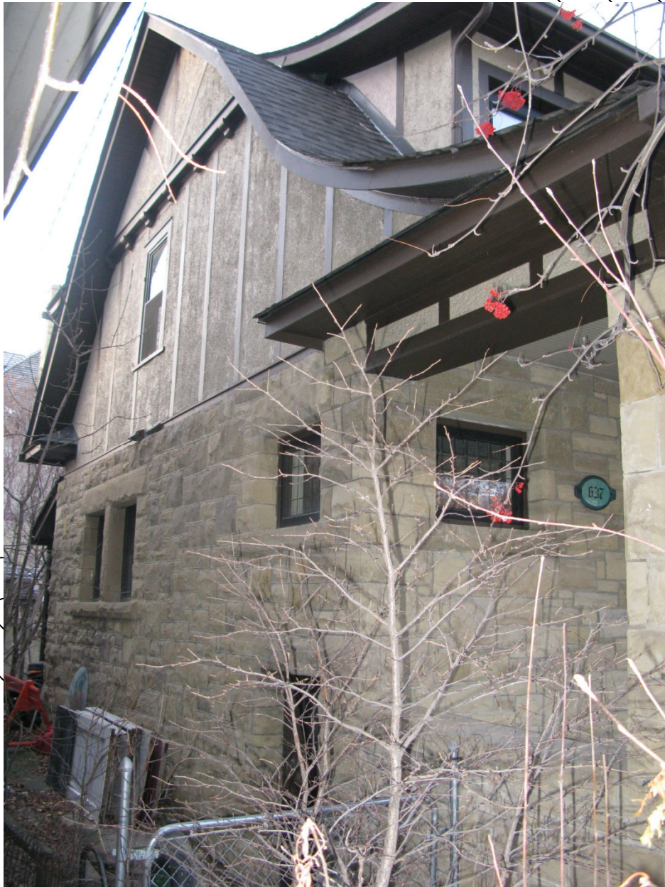
(Photo 3.2: oblique view from the North of East Façade)
