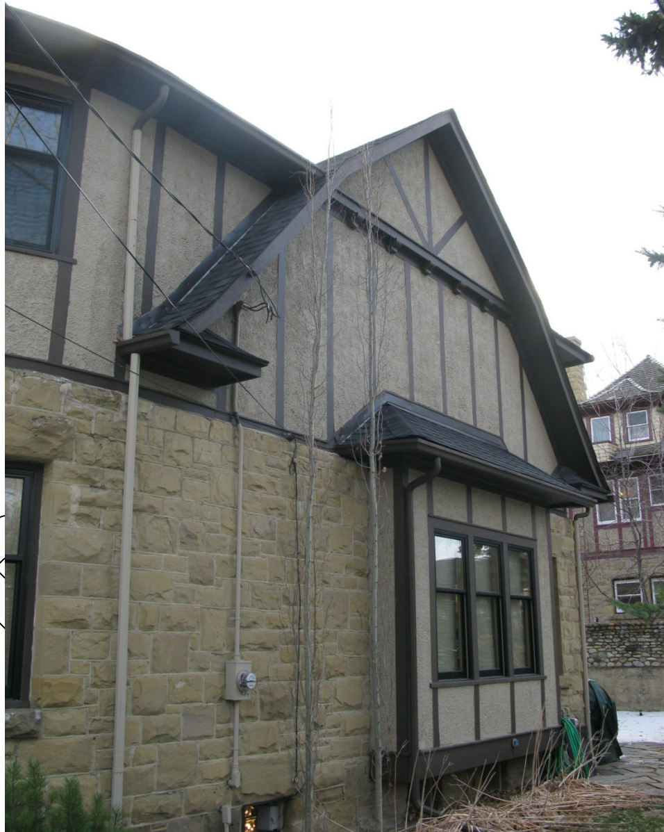
(Photo 4.2: Oblique view from the North of the West Façade.)
