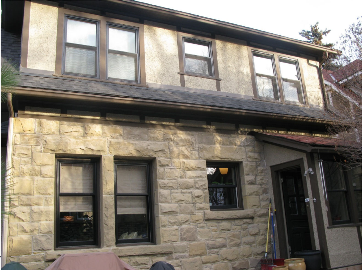
(Photo 5.2: view of South Façade
