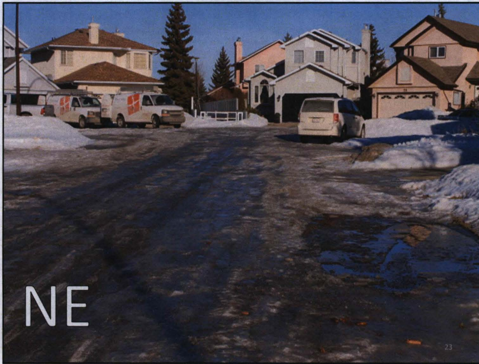
An ice covered road with minimal rutting in the northeast.
