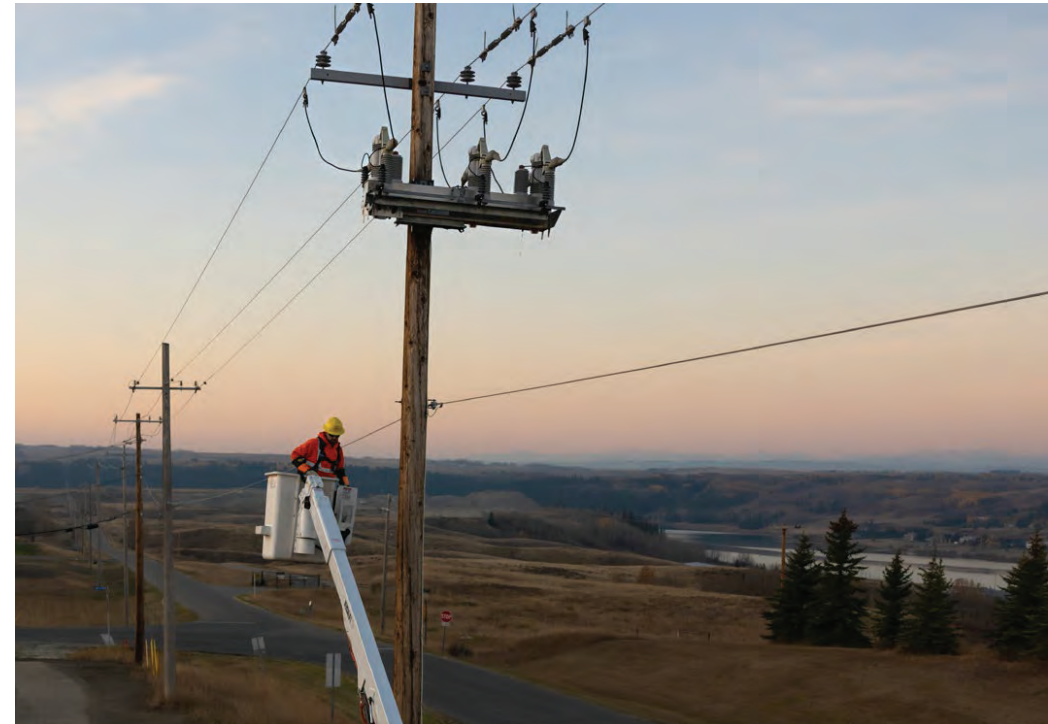
A power systems electrician from ENMAX Power conducting switch maintenance.
