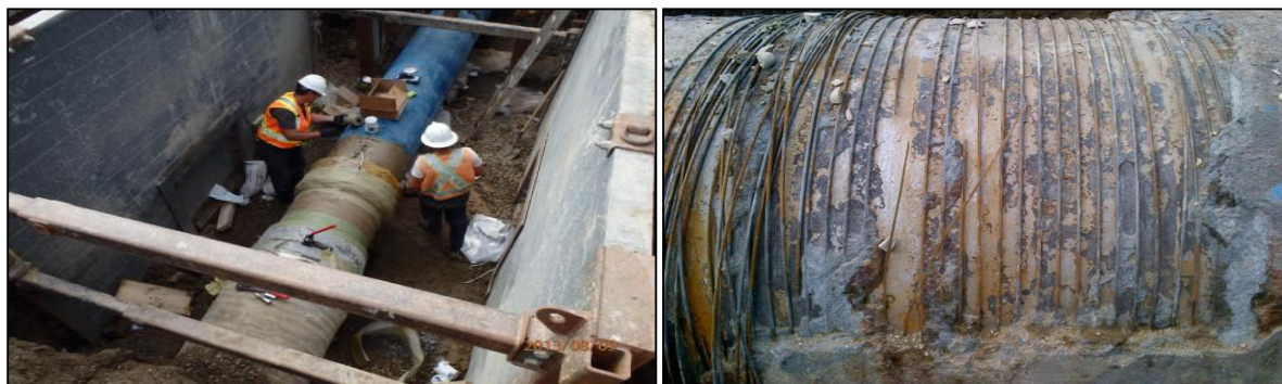
Figure 3b: 68 th Street Feedermain Repair
