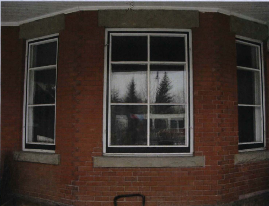
(Photo 2.4: Detail view of the East Façade showing original windows with storm sashes)
