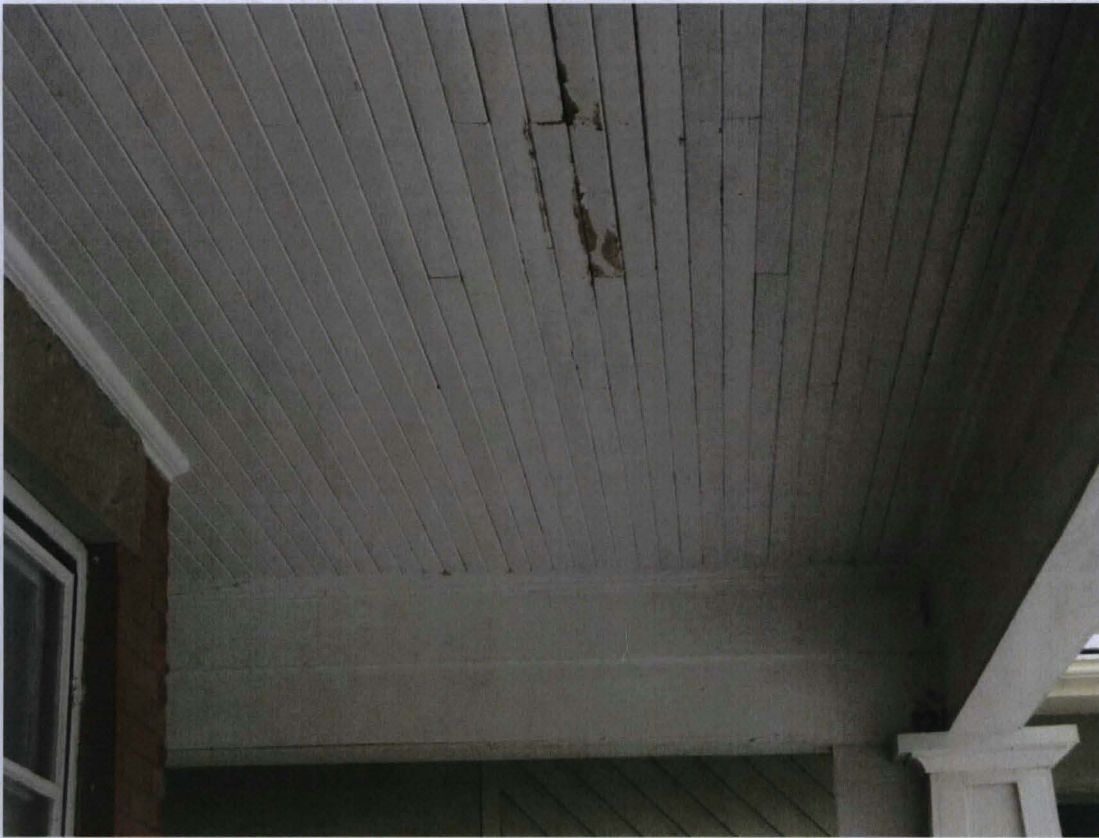
(Photo 2.5: Detail view of the East Façade showing the veranah's frieze and tonge-and-groove ceiling.)
