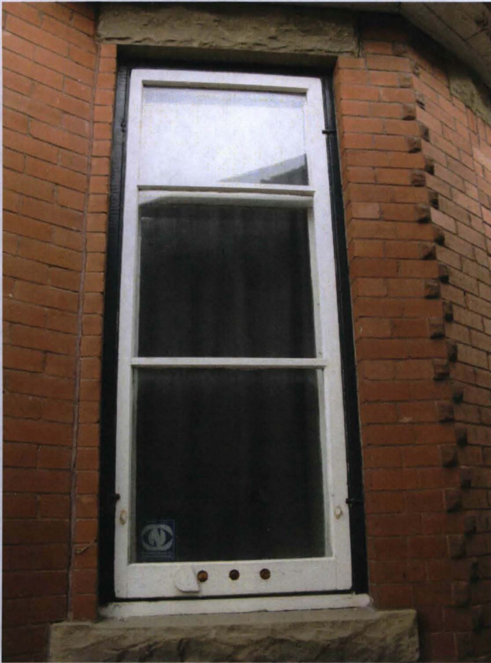
(Photo 4.4: An example of one of the two extant original windows on the North Façade – with storm sash.)
