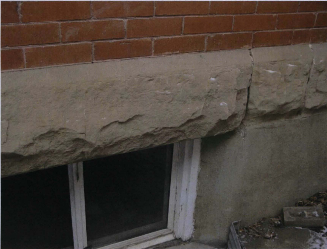
(Photo 3.3: Detail view showing an example of the rough-faced sandstone water table on the South Façade and which also surrounds the West and North Facades.)
