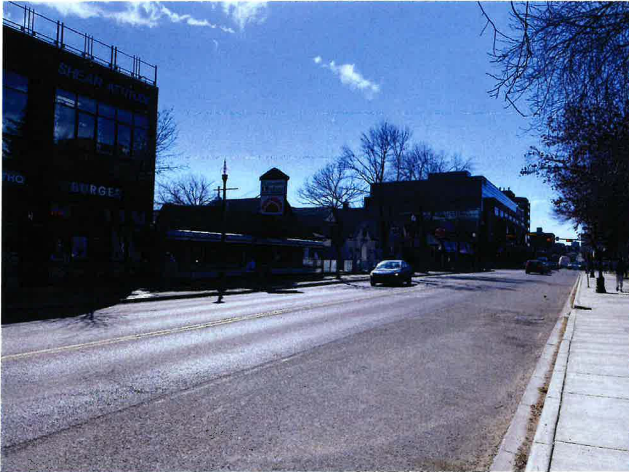
Looking West along 17 Ave SW
