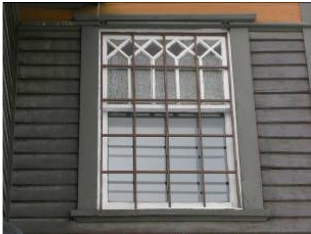
(Photo 1.6: Hung-sash window with a single-pane lower sash and a patterned upper sash with textured and stained glazing (second storey) and corniced casing)
