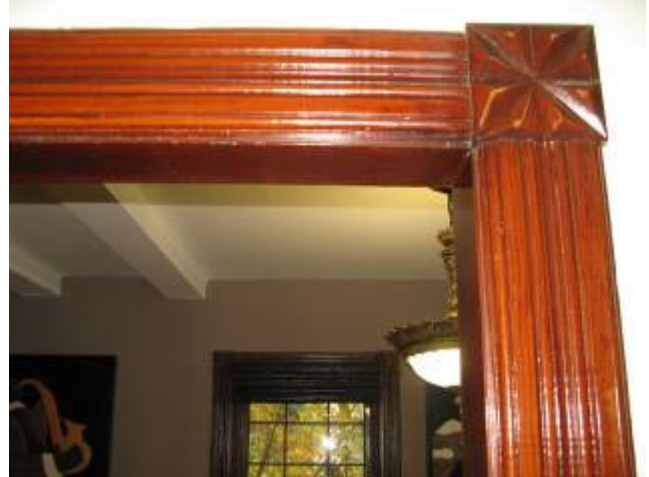
(Photo 6.11: Example of the second-floor window and door casings – note some casings retain a varnish finish while some are painted)
