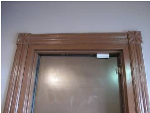
(Photo 6.12: Example of the second-floor window and door casings – note some casings retain a varnish finish while some are painted)
