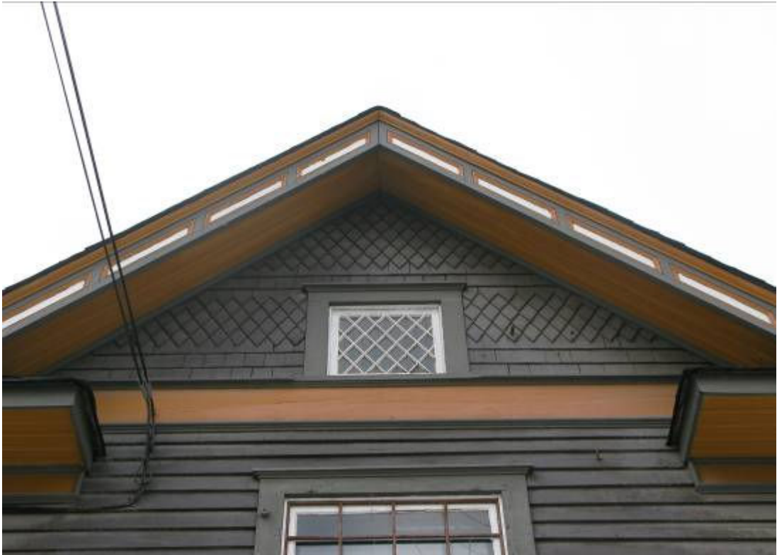
(Photo 1.3: Gable cladding showing alternating courses of regular and diamond-shaped shingles with frieze band below)
