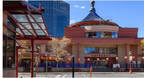
Calgary Chinese Cultural Centre, constructed in 1992
