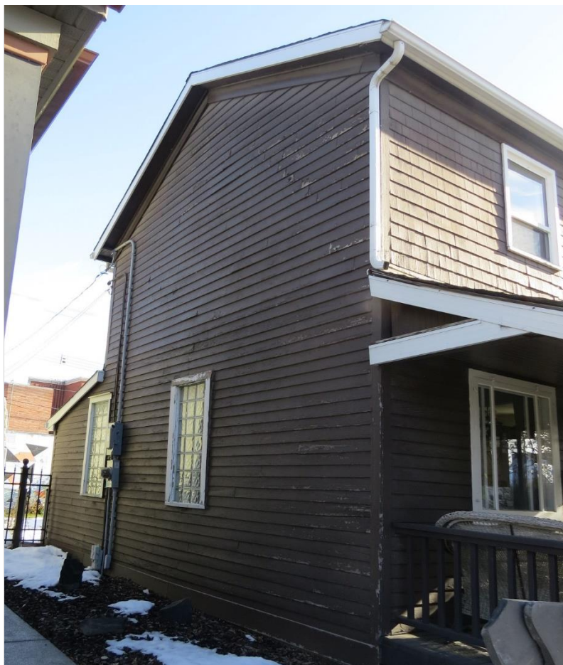
(Image 2.10 – South and west façades, showing beveled wood siding, and wood shingle cladding on south façade second storey)
