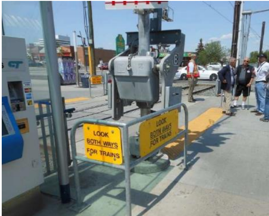
Figure 7: Tactile warning strip at Chinook Station
