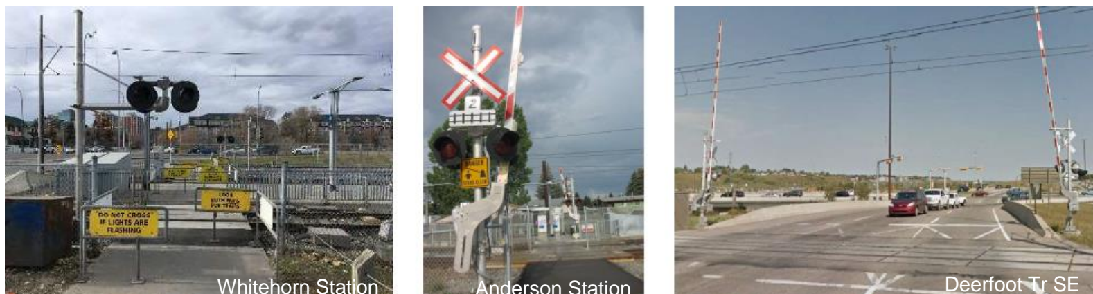
Figure 1: (left) flashing lights, bells and besteads; (middle) automatic pedestrian gate arm, flashing light and bells; (right) automatic vehicle gate arms
