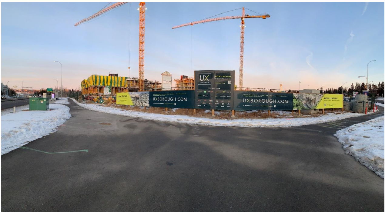
Figure 6: Pathway User Looking West – Photo January 2023
