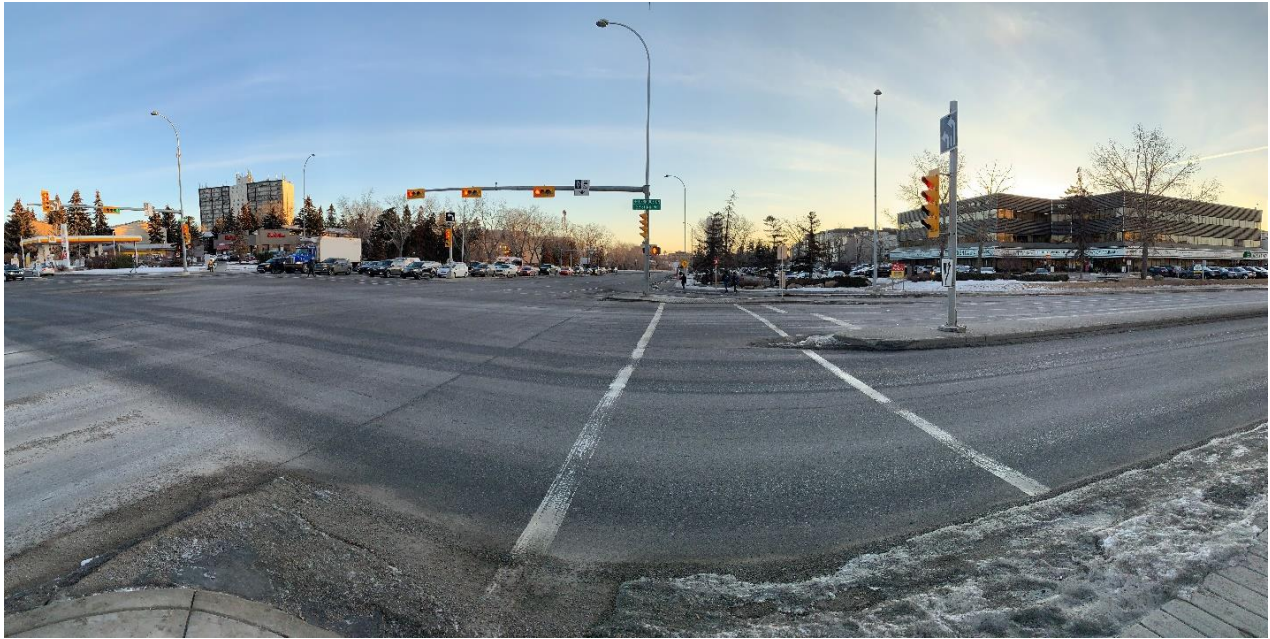
Figure 5: Pathway User Looking East– Photo January 2023
