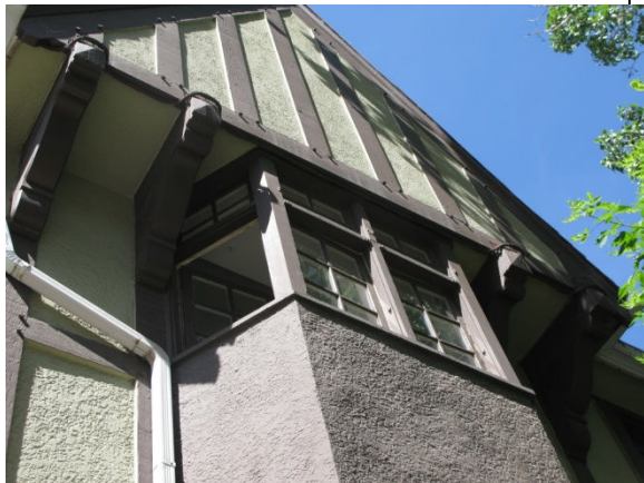
(Photo 1.4: overhanging gable with exposed beam and bracket mouldings)
