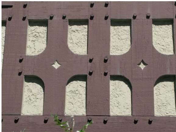
(Photo 1.3: an example of the pegged half timbering)
