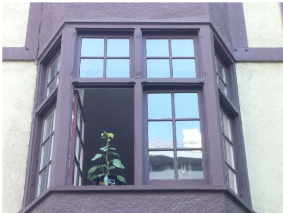
(Photo 1.9: an example of the three-storey bay windows containing six-pane wooden casement sashes and four-pane transom lights)
