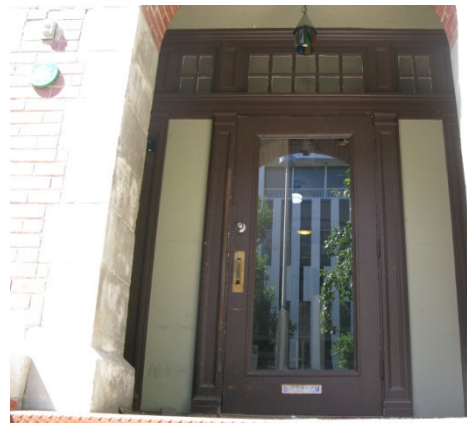
(Photo 1.10: main entrance interior wooden doorway assembly consisting of a single, glazed wooden door surrounded by multi-pane transom lights and sidelights)
