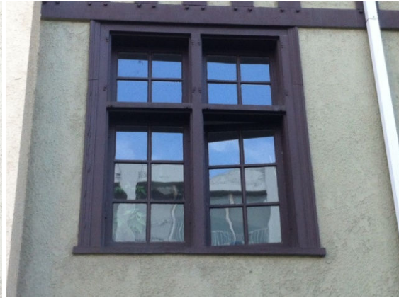
(Photo 1.8: an example of wooden, casement-sash six-pane windows with four-pane transom lights)
