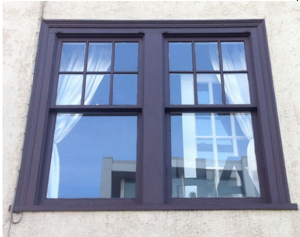
(Photo 1.7: an example of two-part, wooden, hung-sash windows with six-over-one profiles)
