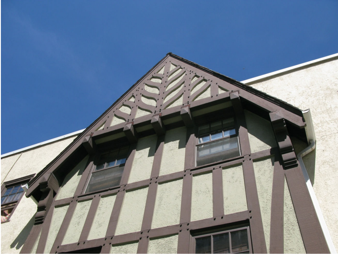
(Photo 3.3: South Façade – detail view of the pegged half timbering with gable overhang and associated exposed beam and bracket mouldings)
