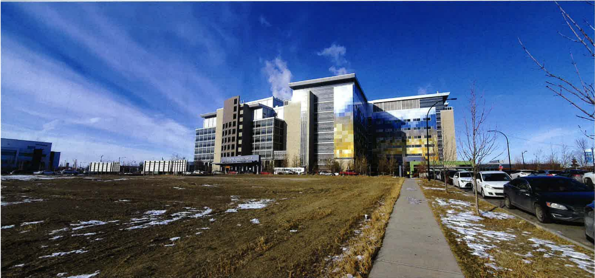
View of the South Health Campus looking
