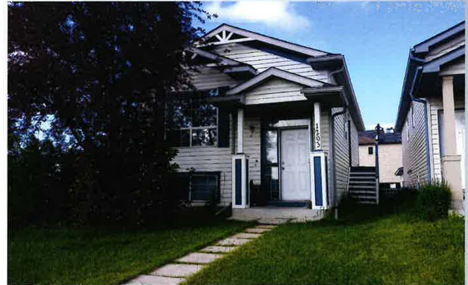
1203 Martindale Blvd NE viewed from Martindale Blvd NE
