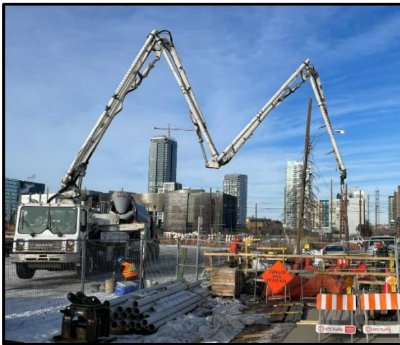
Enmax vault installation in Beltline East
