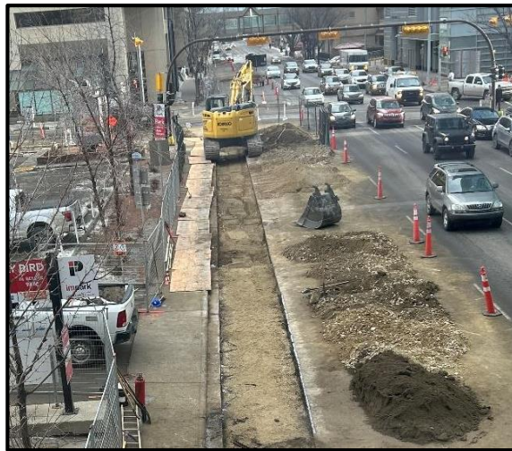
Telus duct bank installation along 4 Ave SW
