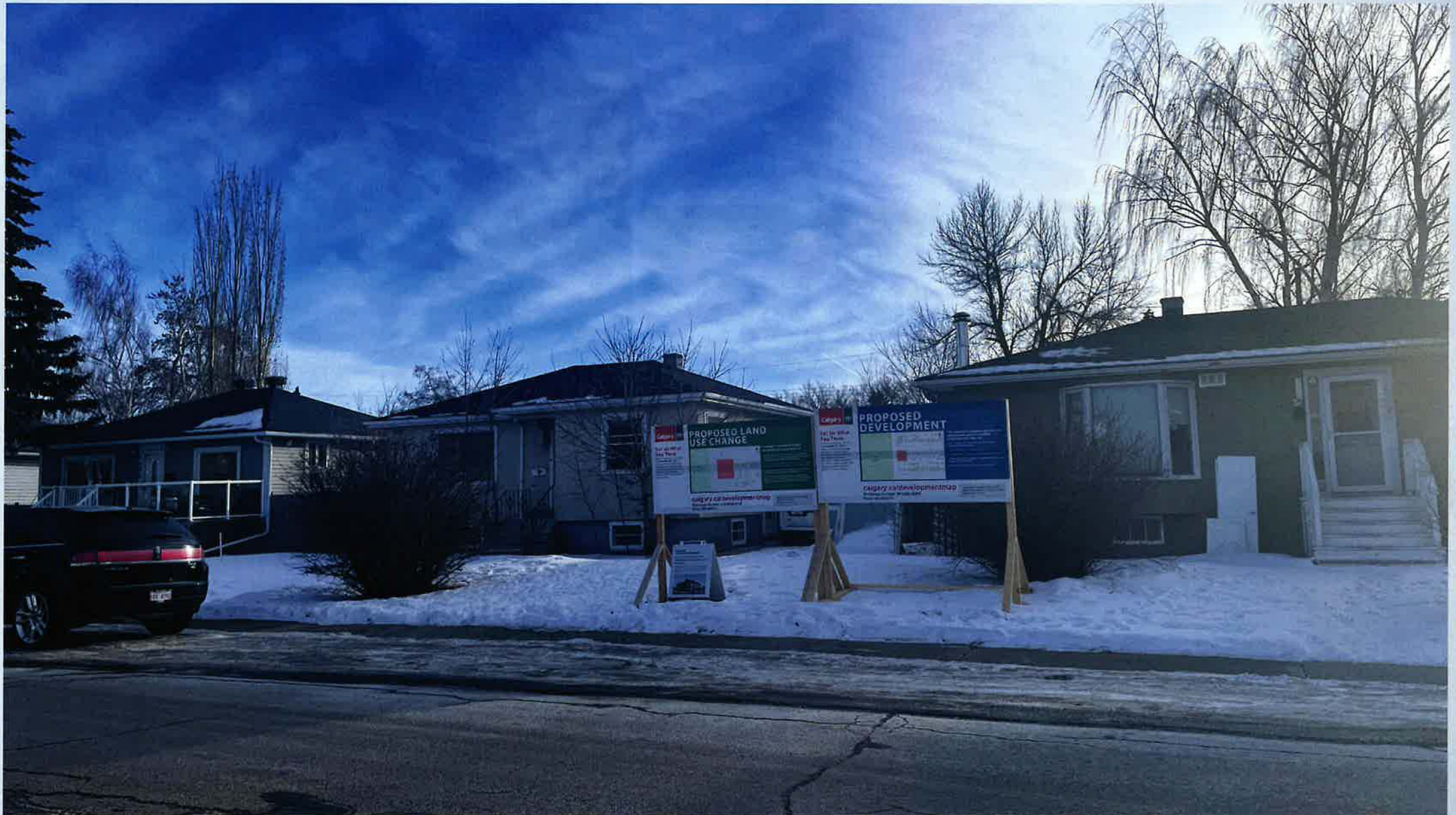
North facades – from 35 Avenue looking south
