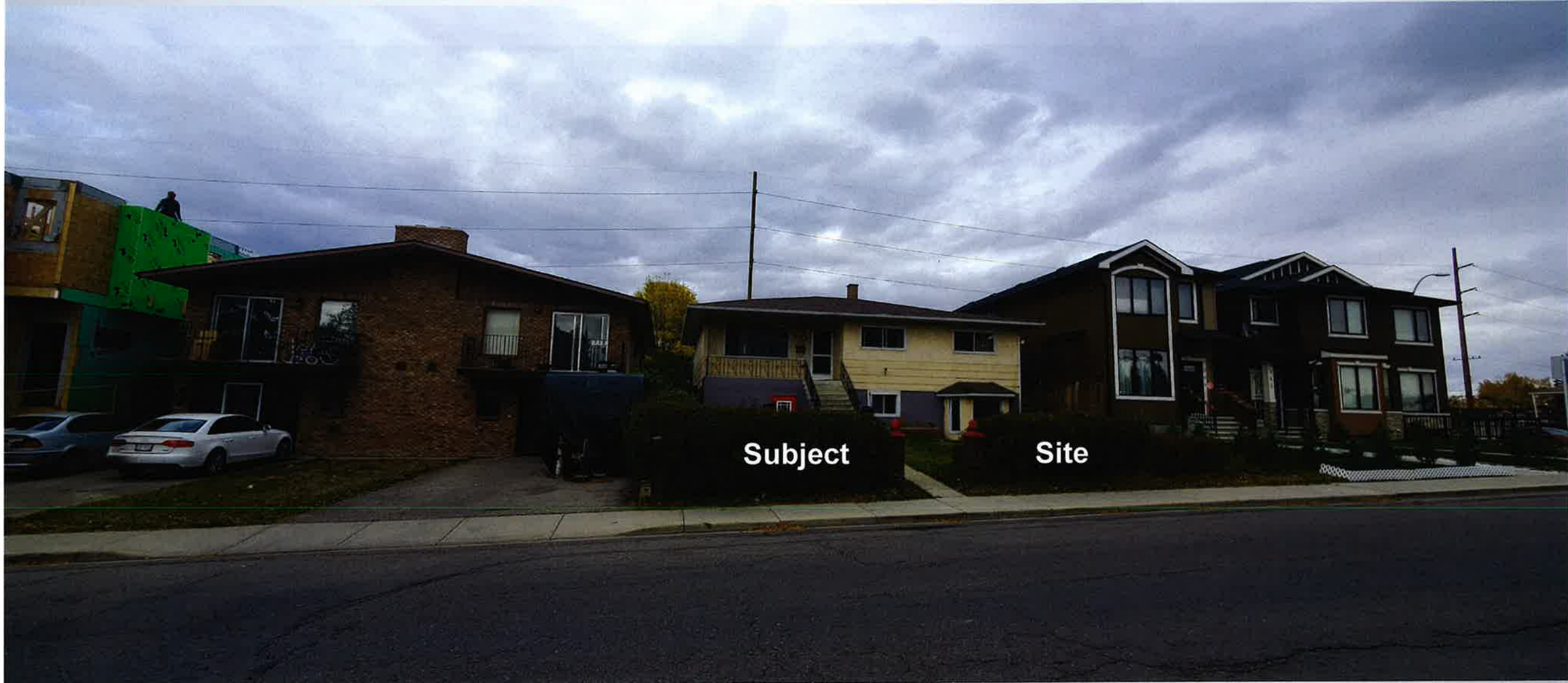
View of the Subject Site looking North
