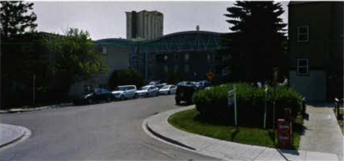
VIEW FROM SITE LOOKING SOUTHEAST TOWARD SAIT
