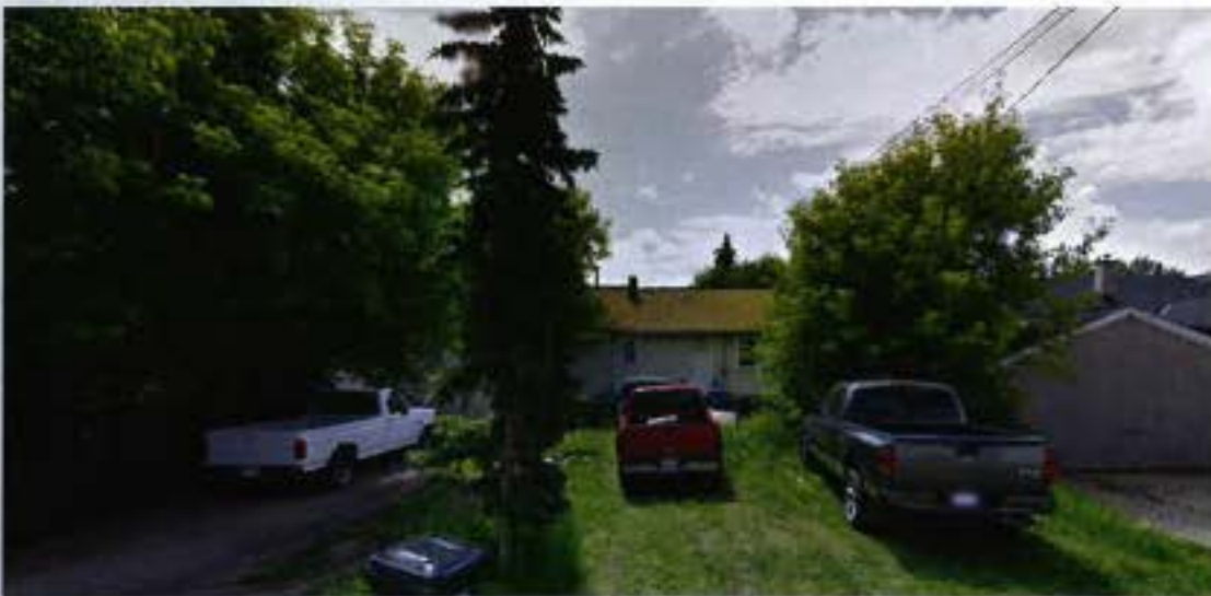
1308 – 17 Avenue NW viewed from the lane
