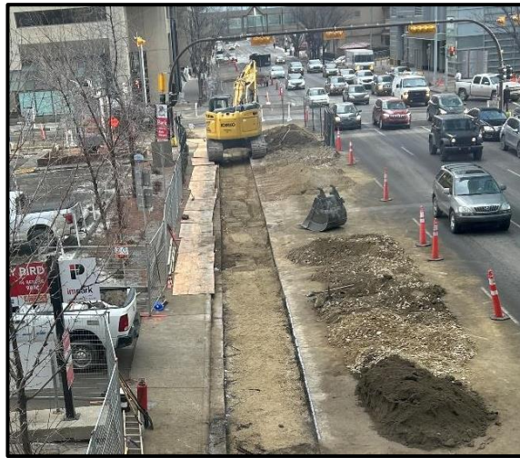
Telus duct bank installation along 4 Ave SW
