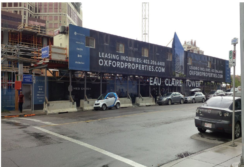
Photo 2 Protective Frame on Sidewalk adjacent to Eau Claire Tower on 3 Avenue SW
