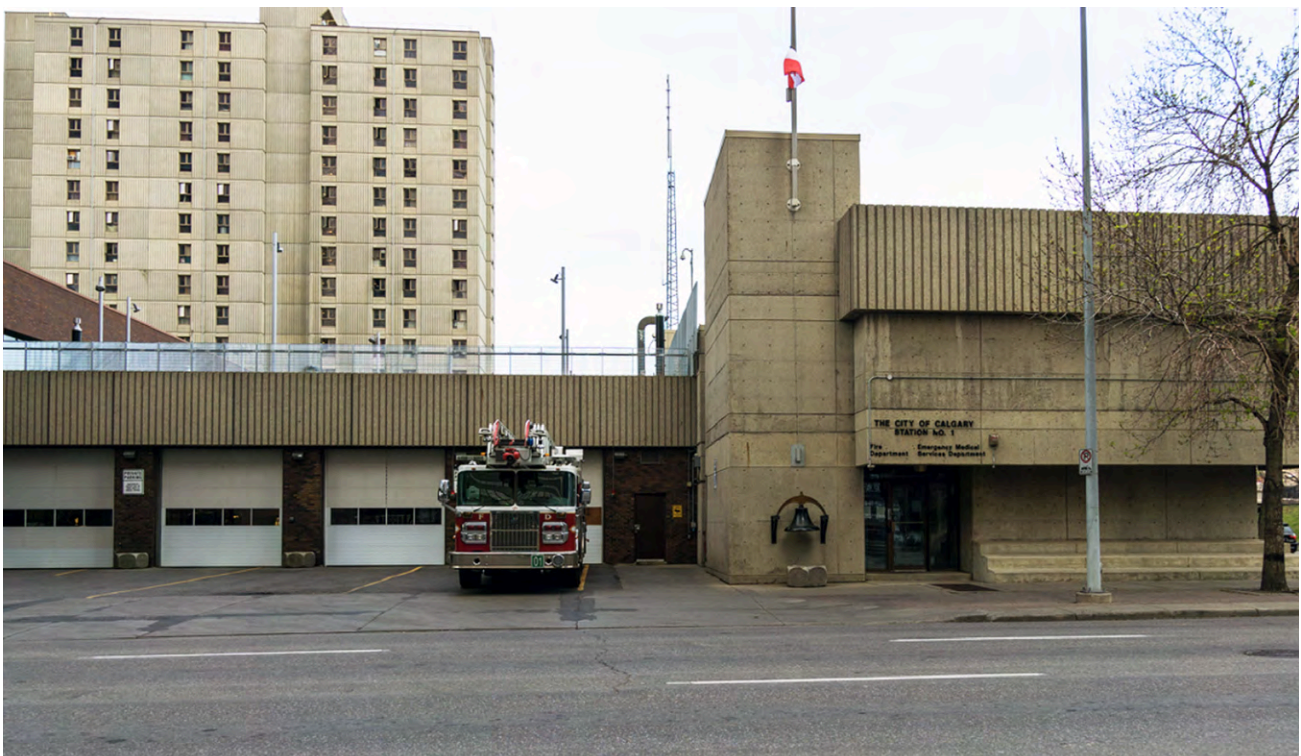
Existing Fire Station No. 1 450 1 ST SE
