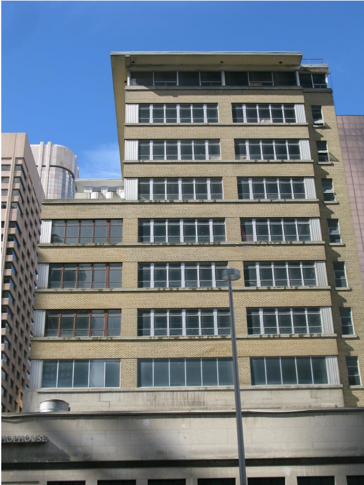
(Image 3.1: View of east façade flat roofs (terraces) where the building steps back at the eighth and eleventh storeys, with deep overhanging eaves at the eleventh storey penthouse, and original rooftop mechanical and elevator house forms, buff-coloured brick spandrel panels framing storeys four through eight)
