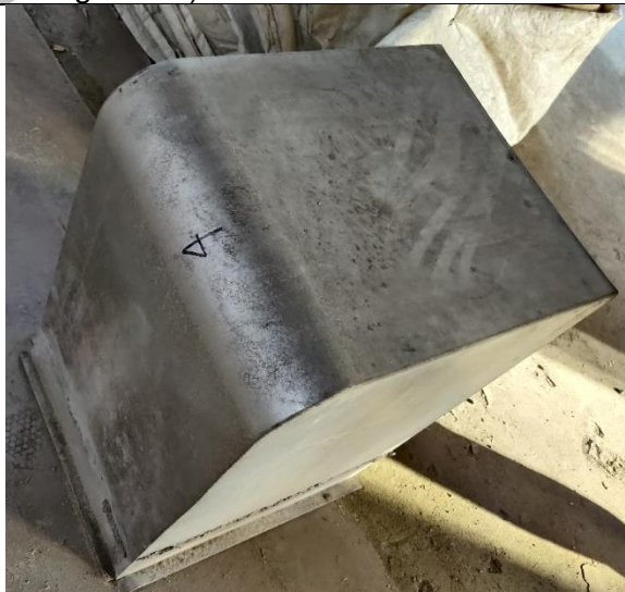
(Image 1.19: 2022 close-up photo of top cap for aluminum pilaster. Deconstructed from its original placement, it will be returned to its original location and configuration)
