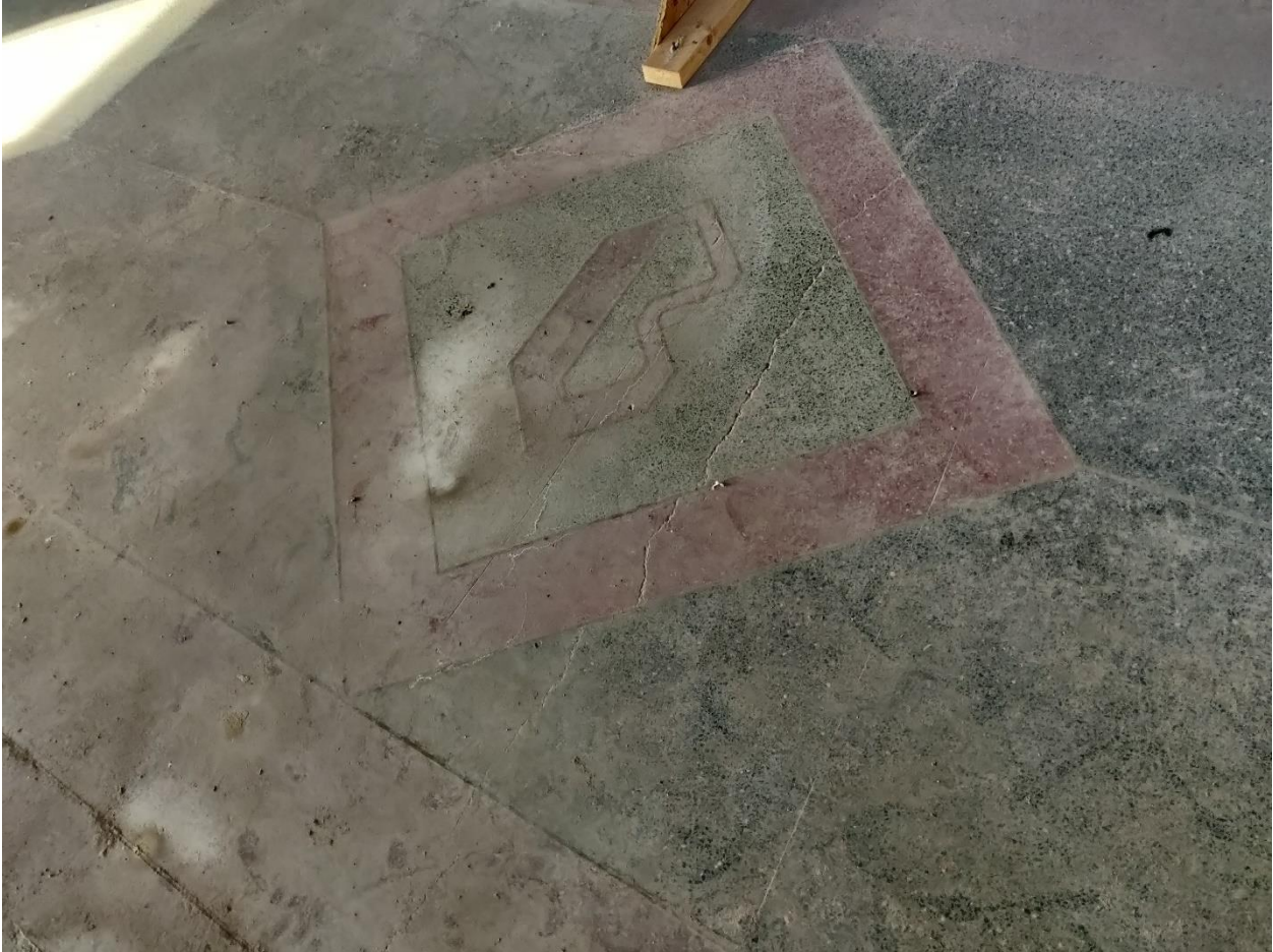
(Image 5.2: Detailed view of terrazzo flooring with brass inlay and 'B' formed in the centre of elevator lobbies from floors two through five, and seven through ten, including re-created sixth storey terrazzo floor )
