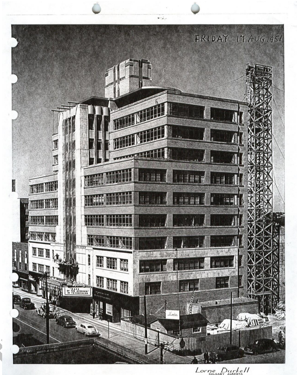
(Image 1.2: 1951 photo showing oblique view of south façade with deep overhanging eaves at the eleventh storey penthouse, and original rooftop mechanical and elevator house forms, geometric-patterned stone banding on elevator house at the rooftop). Photo Credit: Daniel Barron
