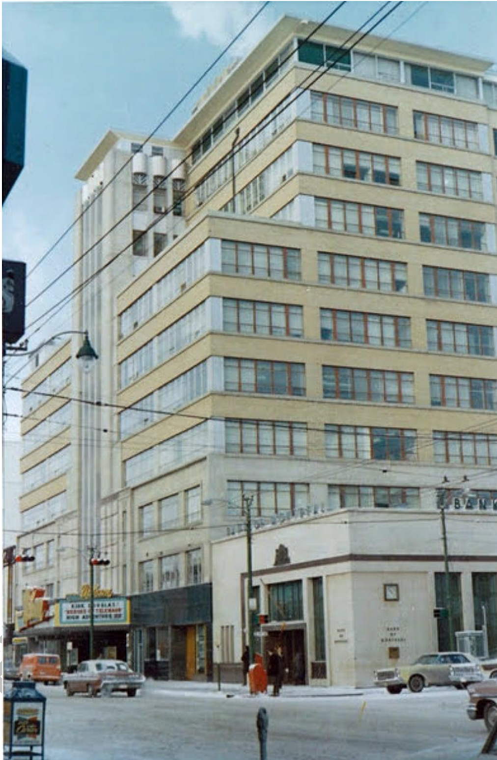
(Image 3.4: 1966 photo showing oblique view of Barron Building from southeast corner showing building stepback at the eighth and eleventh storey with deep overhanging eaves at the historic eleventh storey penthouse, expanded from original 1952 form and massing) Photo Credit: Daniel Barron
