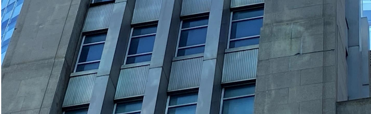
(Image 1.7: Stylized aluminum-clad pilasters on central frontispiece with scalloped aluminum cladding details at spandrel panels from storeys two through ten)
