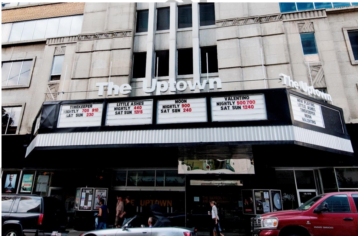
(Image 1.5: Black granite tile sheet cladding framing the first storey, and honed Tyndall limestone windowsills, copings, spandrel panels and ornaments for storeys two through four)
