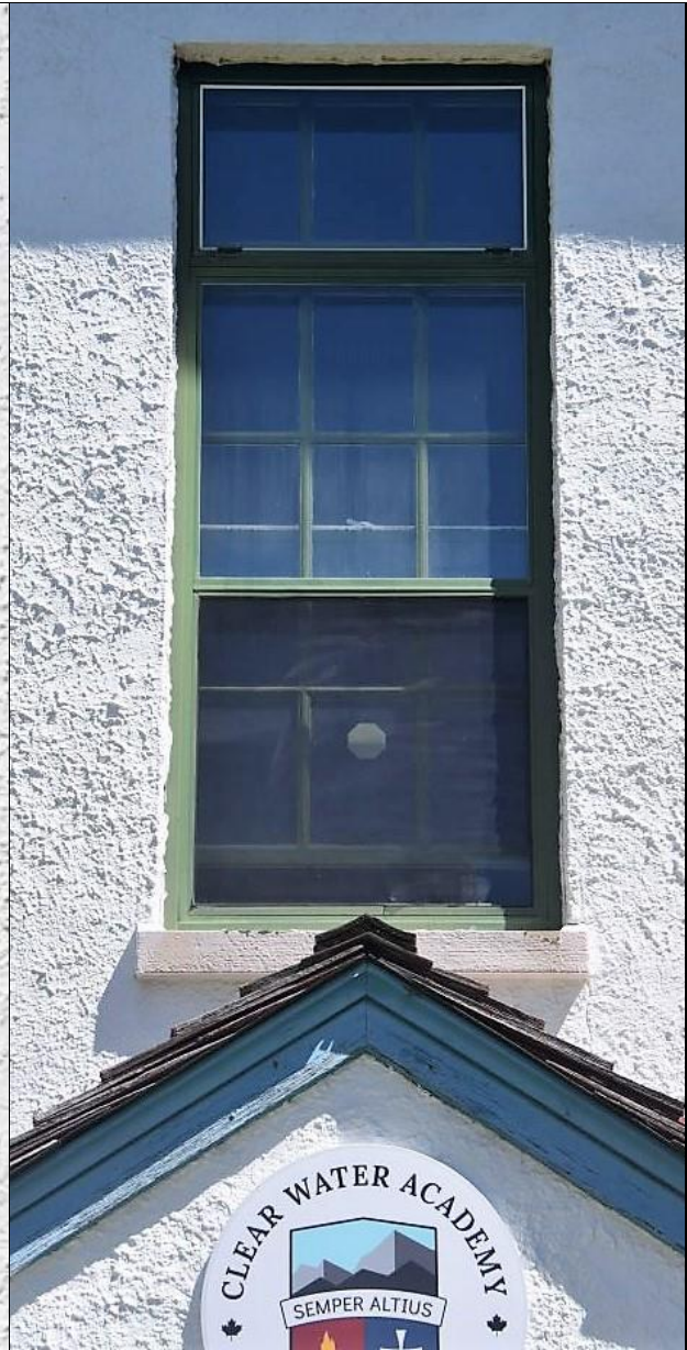
Image 2.17: Example of typical nine-over-six pane window, stone plain lug sill.
