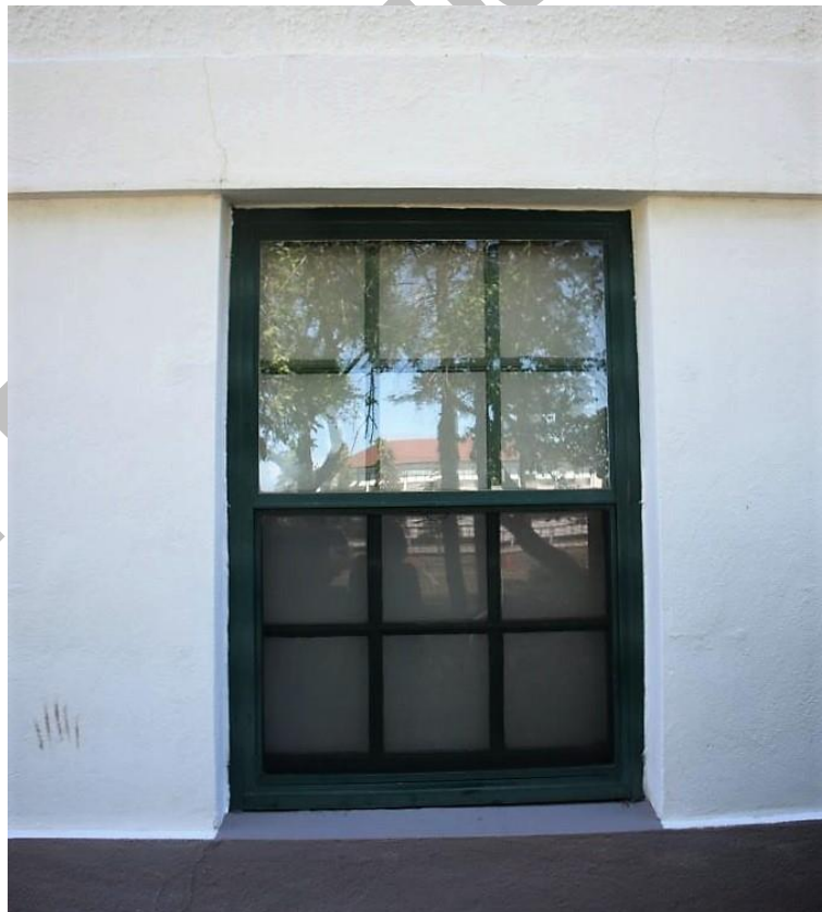
(Image 2.15: Example of typical six-over-six pane window on basement level)
