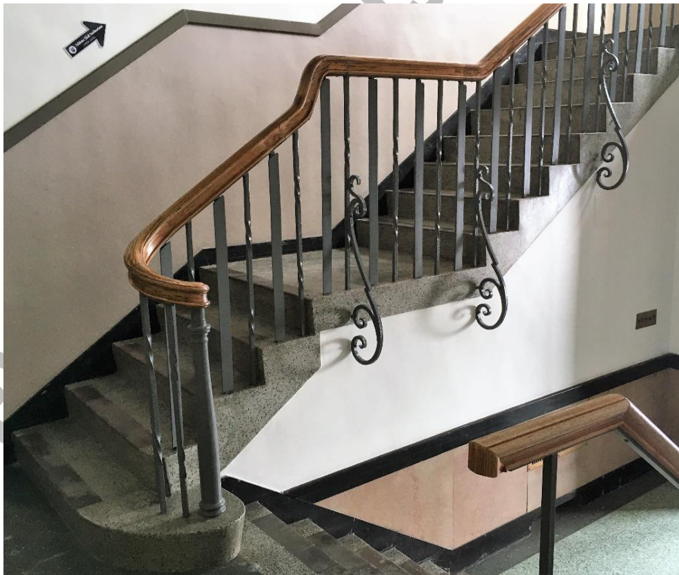
(Image 3.3: Lower portion of double return main staircase, cast-iron newel post, ornamental wrought iron balustrade and decorative bracket supports)
