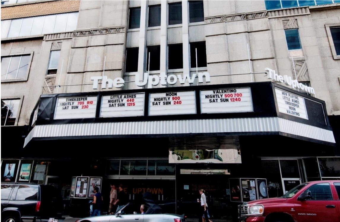
(Image 1.5: Black granite tile sheet cladding framing the first storey, and honed Tyndall limestone windowsills, copings, spandrel panels and ornaments for storeys two through four)
