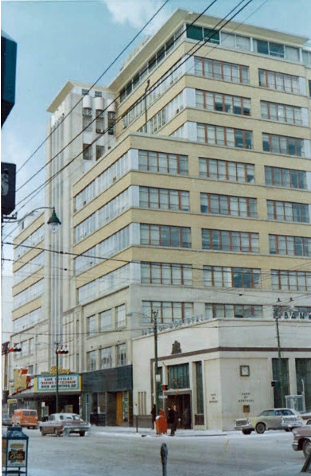
(Image 3.4: 1966 photo showing oblique view of Barron Building from southeast corner showing building stepback at the eighth and eleventh storey with deep overhanging eaves at the historic eleventh storey penthouse, expanded from original 1952 form and massing) Photo Credit: Daniel Barron
