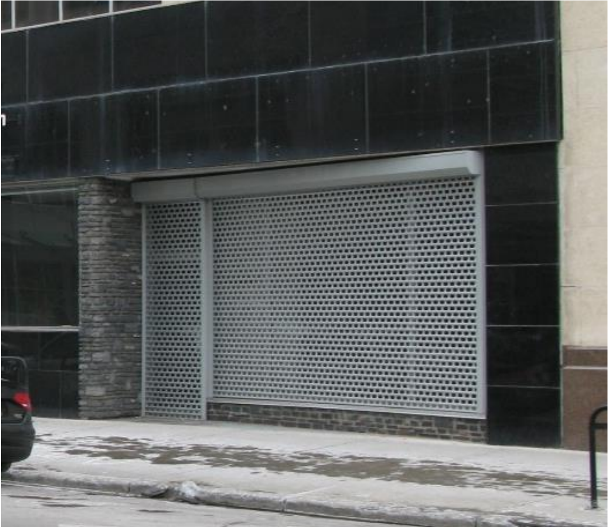
(Image 1.10: Detailed view of black granite cladding on the angled storefront at the southeast façade. View of junction of black granite and Tyndall limestone)
