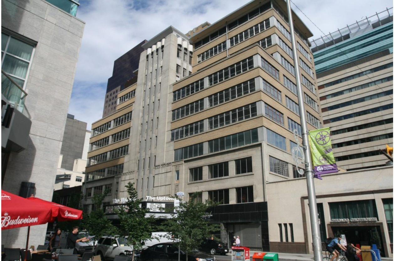
(Image 3.2: View of east façade flat roofs (terraces) where the building steps back at the eighth and eleventh storeys, with deep overhanging eaves at the eleventh storey penthouse, and original rooftop mechanical and elevator house forms, buff-coloured brick spandrel panels framing storeys four through eight)
