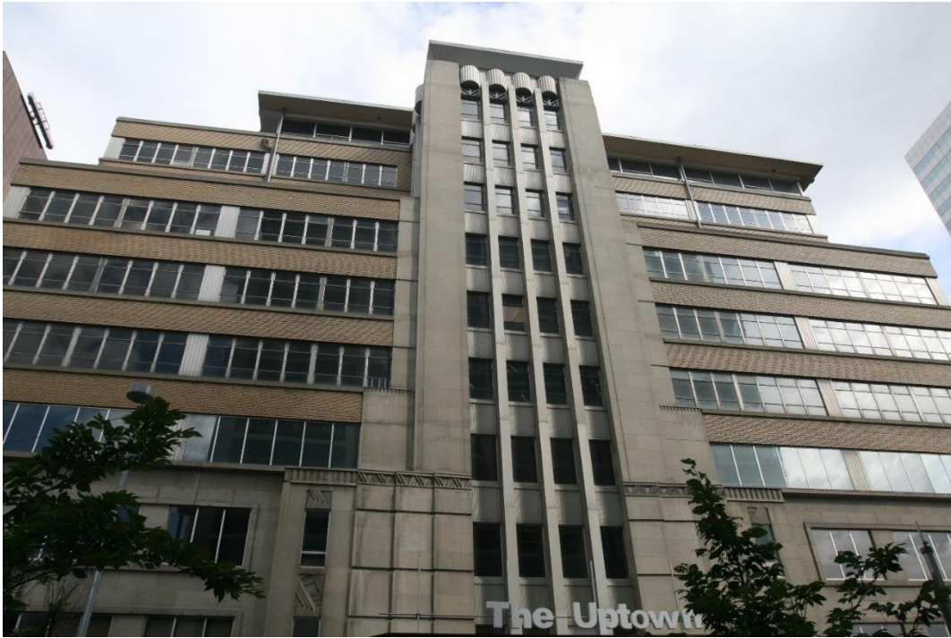
(Image 1.6: South façade photo showing honed Tyndall limestone vertical central frontispiece on storeys two through eleven, scalloped aluminum cladding details at spandrel panels on central frontispiece rising from storeys two through ten, four vertical bands of windows on central frontispiece rising from storey two through ten, stylized aluminum-clad pilasters on central frontispiece from storeys two through ten, curved, stylized aluminum panels curved aluminum panels with scalloped profile and Art-Moderne ornamentation displaying carved, low-relief panels with geometric-patterned stone detail at the eleventh storey)
