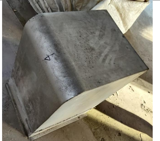
(Image 1.19: 2022 close-up photo of top cap for aluminum pilaster. Deconstructed from its original placement, it will be returned to its original location and configuration)
