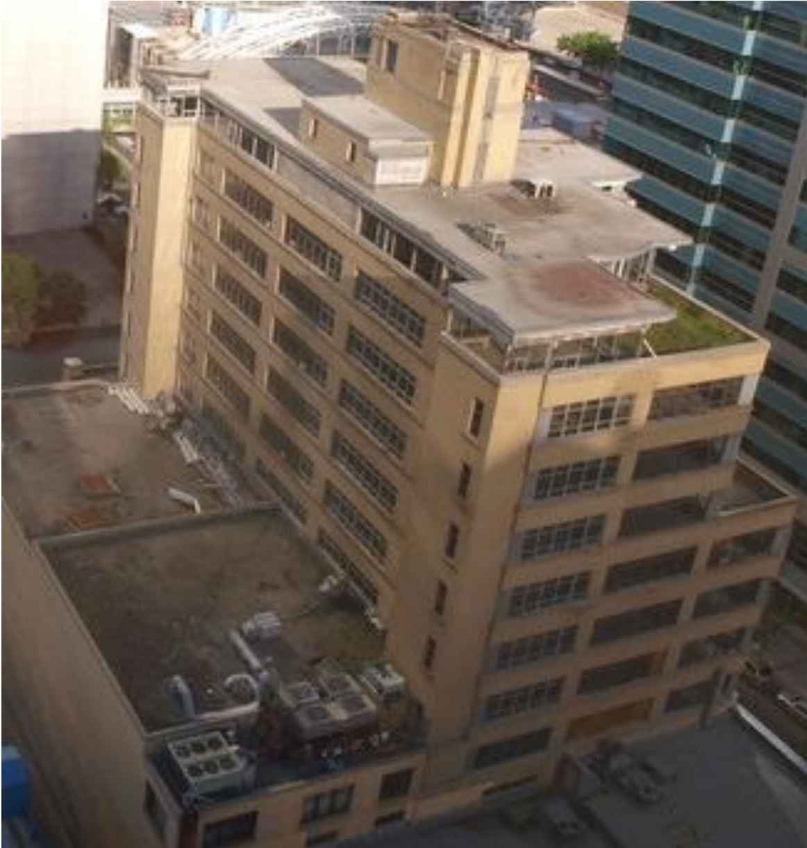
(Image 4.1: Aerial view Barron Building from northwest corner showing building stepback at the eighth and eleventh storey with deep overhanging eaves at the eleventh storey penthouse, and original rooftop mechanical and elevator house forms)
