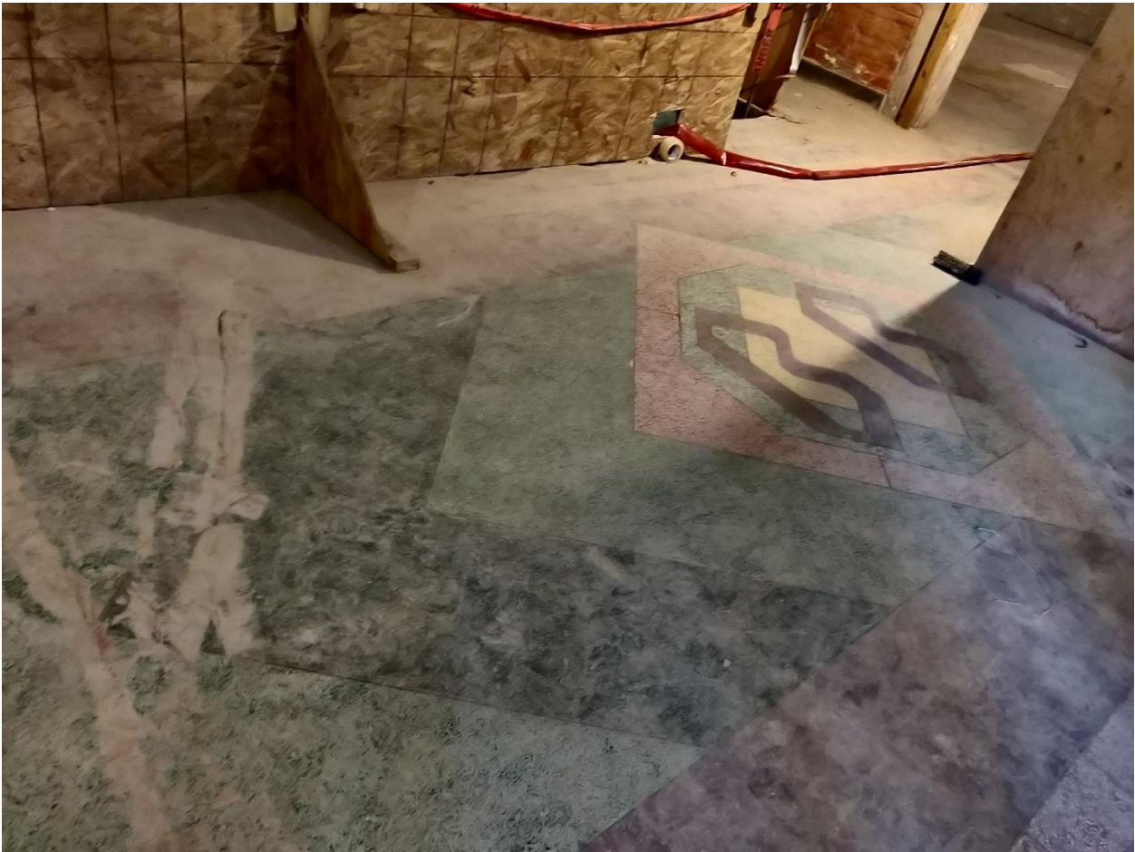
(Image 5.1: View of main floor lobby with ‘BB’ cast into terrazzo flooring)
