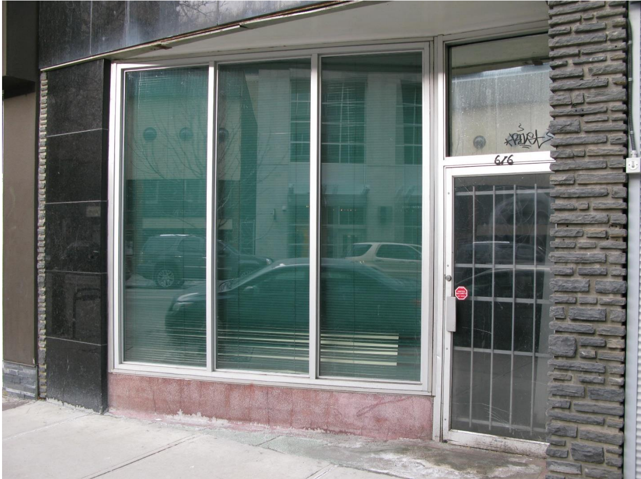
(Image 1.11: Detailed view of black granite cladding on the angled storefront at the southwest façade)
