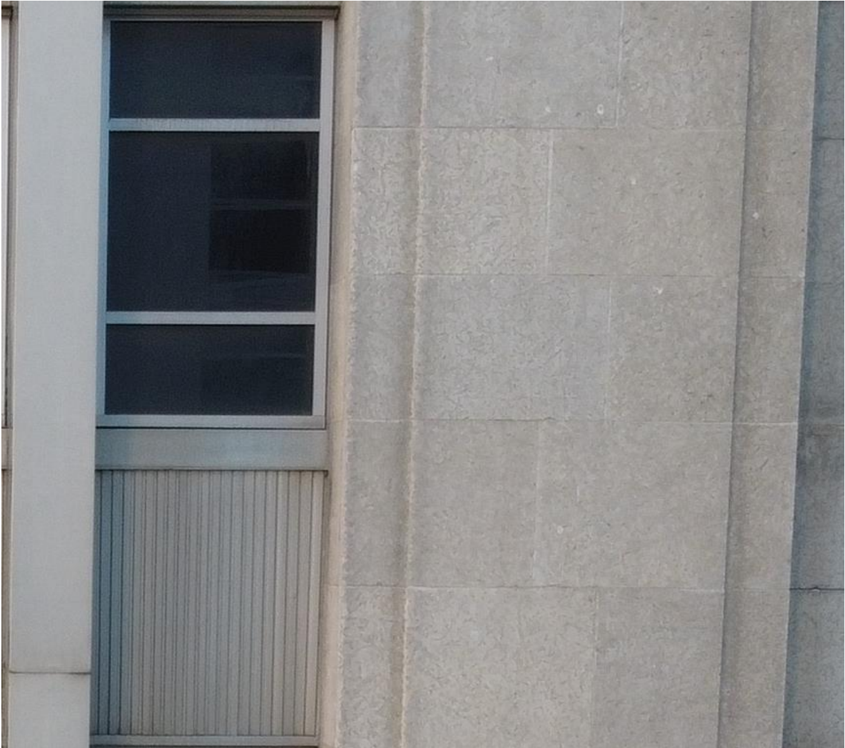
(Image 1.8: Detailed view of central frontispiece's stylized aluminum pilaster on the left, scalloped aluminum cladding details at spandrel panels in the middle and limestone pilaster on the right).
