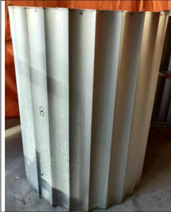
(Image 1.16: 2022 close-up photo of curved, stylized aluminum panel with scalloped profile. Deconstructed from its original placement, it will be returned to its original location and configuration)
