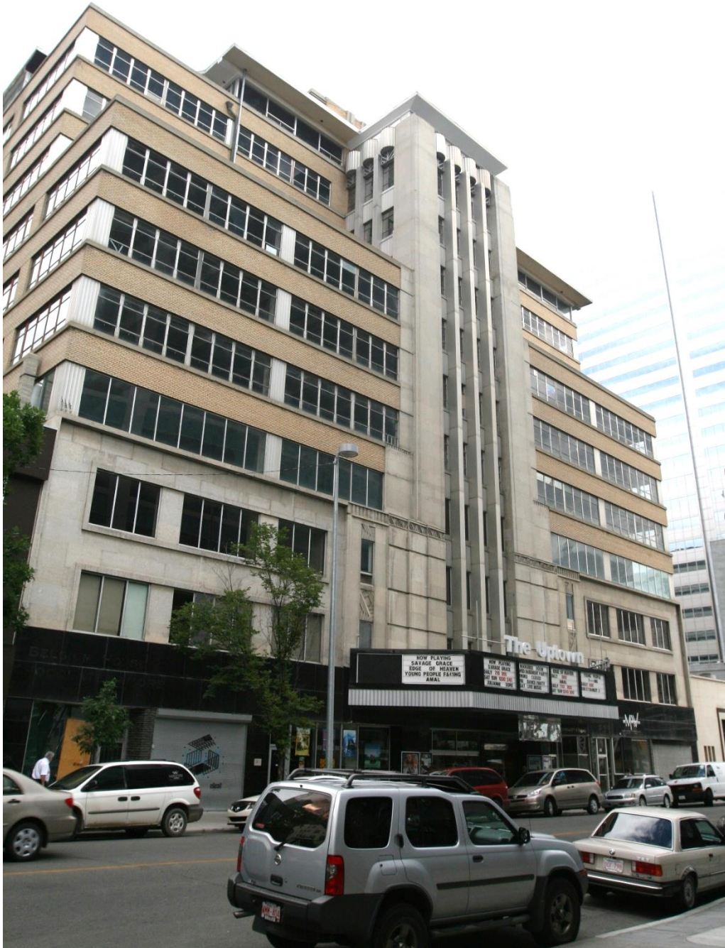
(Image 1.1: Oblique view of south façade showing black granite tile sheet cladding framing the first storey with angled storefronts, concrete tile cladding framing the second and third storeys, buff-colored brick spandrels framing with scalloped sheet aluminum cladding details at corners and in front of the columns from storeys four through ten, with fenestration comprised of ribbon windows from storeys two through eleven)
