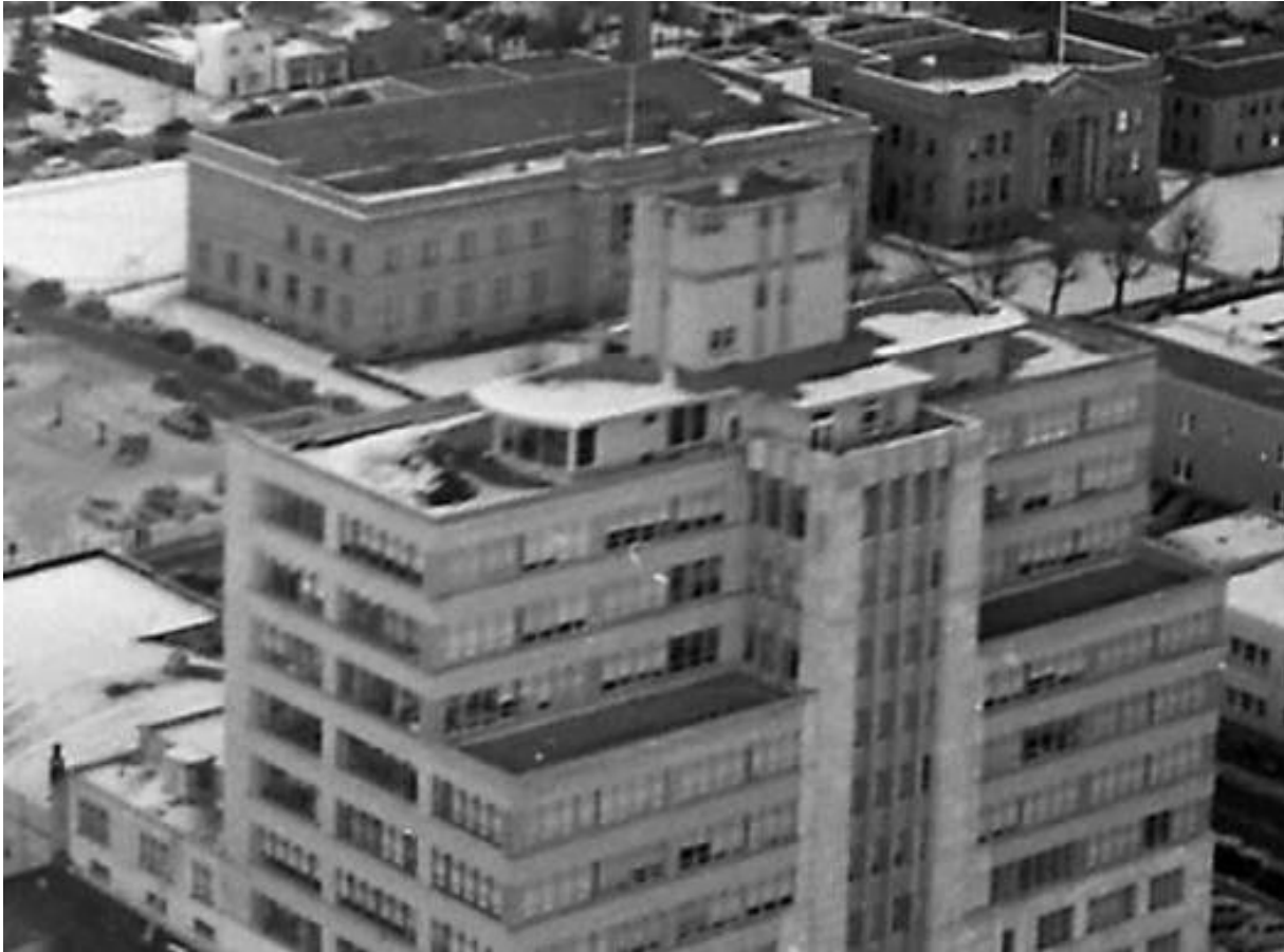
(Image 2.2: 1951 photo showing aerial view of Barron Building from southwest corner showing building stepback at the eighth and eleventh storey with deep overhanging eaves at the eleventh storey penthouse, and original rooftop mechanical and elevator house forms). Photo Credit: Daniel Barron
