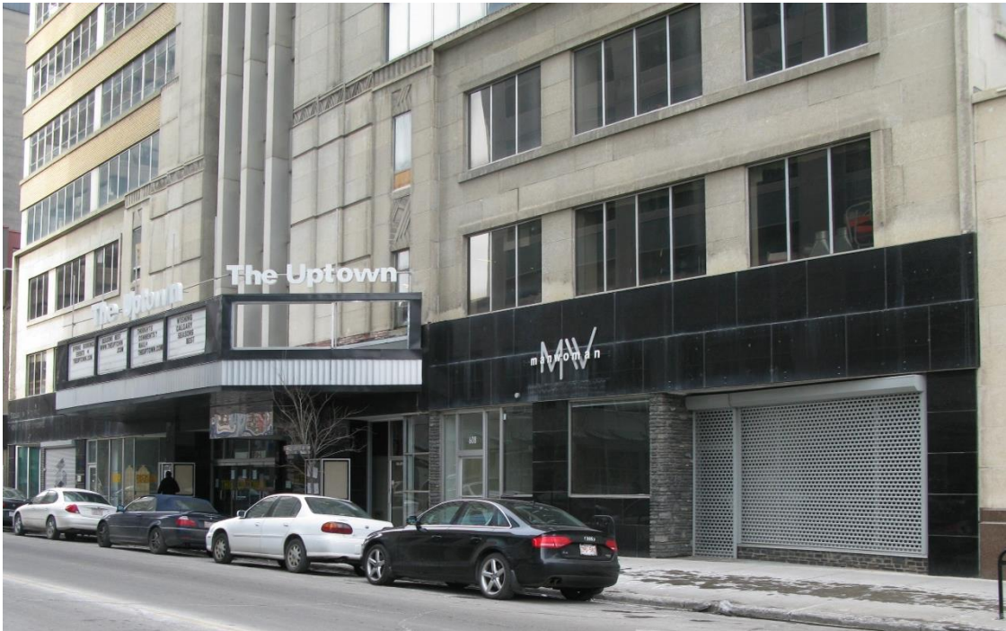
(Image 1.4: Black granite tile sheet cladding framing the first storey with angled storefronts, and honed Tyndall limestone windowsills, copings, spandrel panels and ornaments for storeys two through four)
