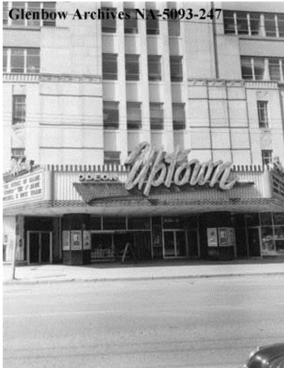
(Image 1.3: 1956 photo showing Black granite tile sheet cladding framing the first storey with angled storefronts, and honed Tyndall limestone windowsills, copings, spandrel panels and ornaments for storeys two through four)
