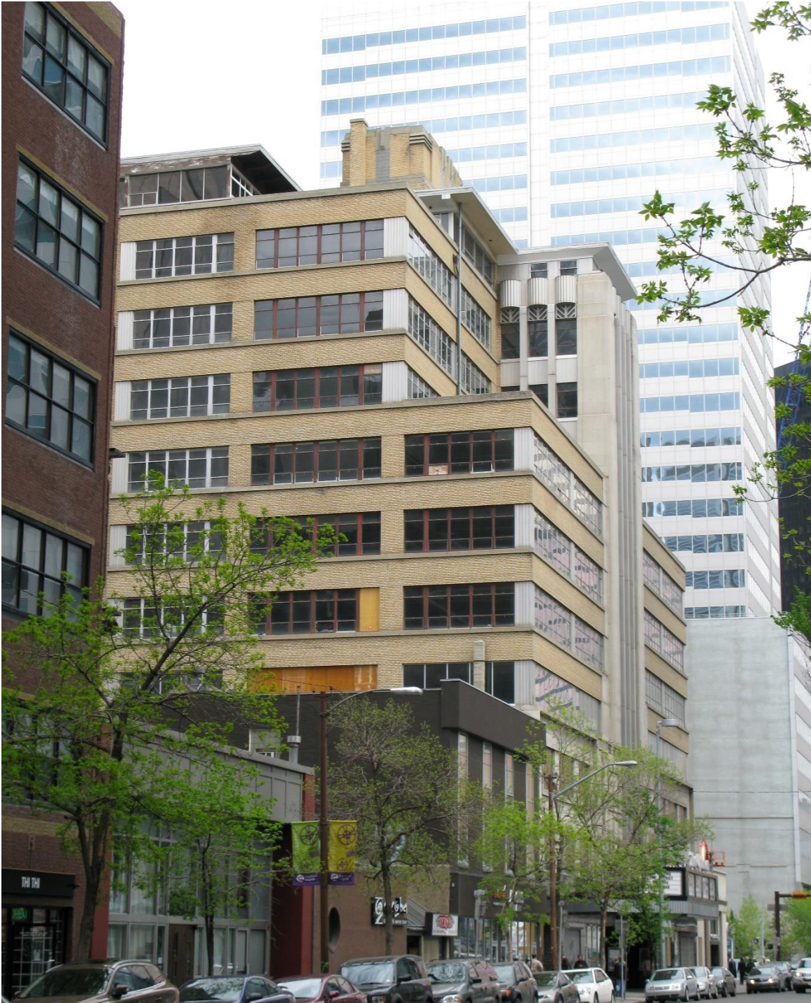
(Image 2.1: Oblique view of the west and south façade showing building stepback at the eighth and eleventh storey, with deep overhanging eaves at the eleventh storey penthouse, and original rooftop mechanical and elevator house forms, fenestration comprised of ribbon windows with scalloped aluminum-panel corners with buff-coloured brick spandrel panels framing storeys four through ten. Curved and stylized aluminum panels with scalloped profile and Art-Moderne ornamentation displaying carved, low relief spandrel panels with geometric-patterned stone detail on the eleventh storey of central frontispiece)
