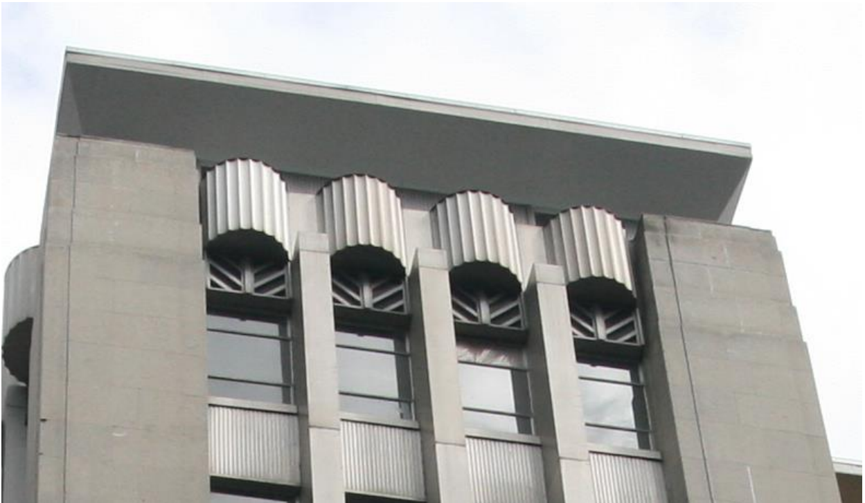
(Image 1.15: curved, stylized aluminum panels with scalloped profile and Art-Moderne ornamentation displaying carved, low-relief panels with geometric-patterned stone detail at the eleventh storey, with deep overhanging eaves)
