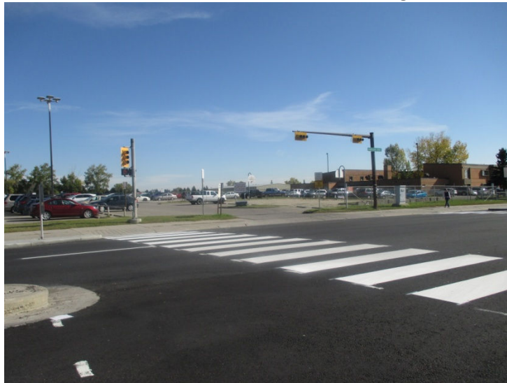
Photo 5 – Ladder Pavement Markings
