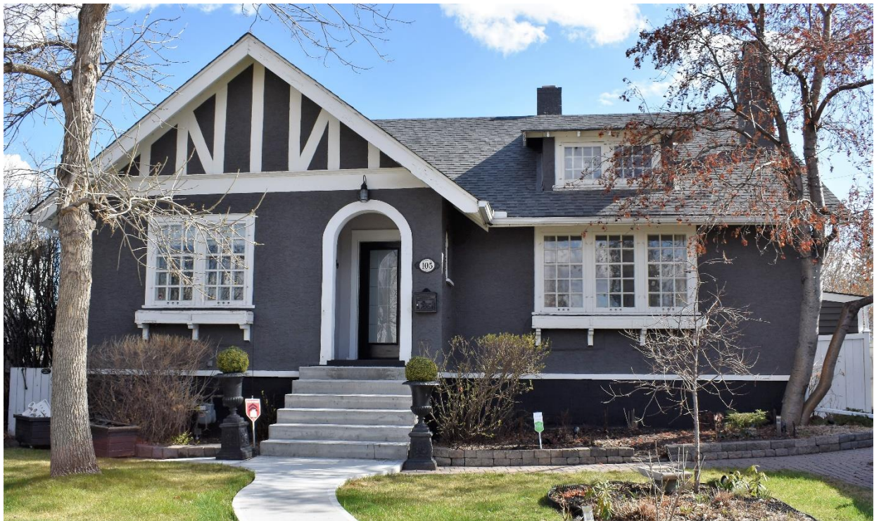
(Image 2.1: North façade)
