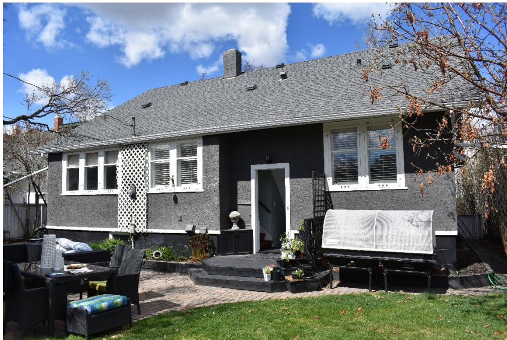
(Image 2.5: South façade)
