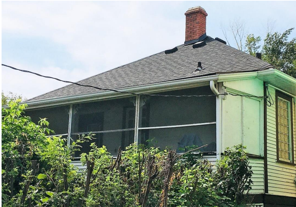
(Image 2.9: Detail of low-pitched shed roof over rear porch)
