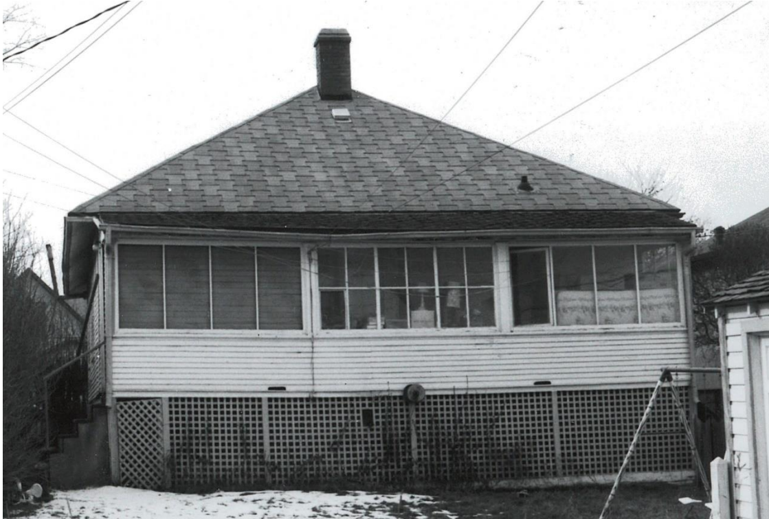
(Image 2.4: East façade with low-pitched shed roof over rear porch, archive image ca. 1984, HS 68461-84-R0130-15)
