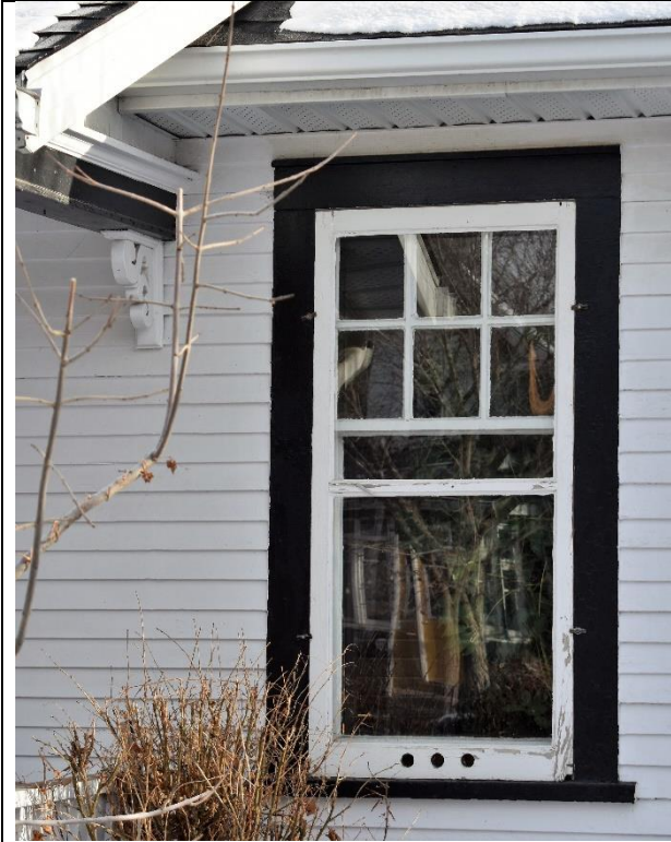
2.10: Detail of typical fenestration, wood side frame and narrow plain lug wood sill
