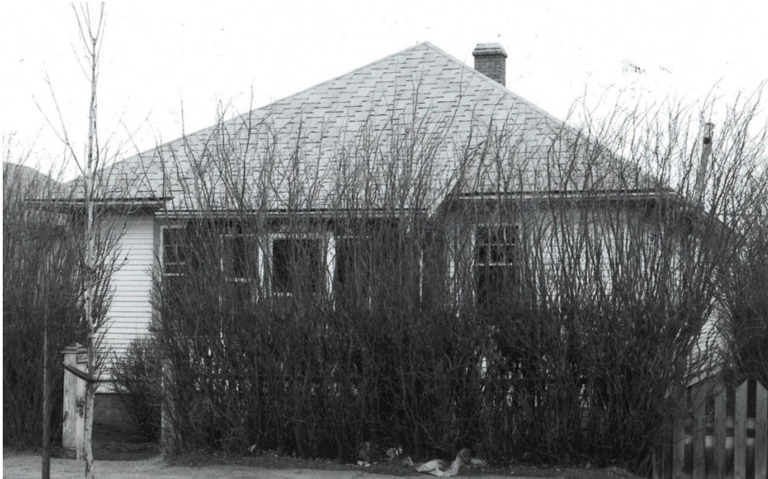
(Image 2.2: West façade, archive image ca. 1984, HS 68461-84-R0130-14)
