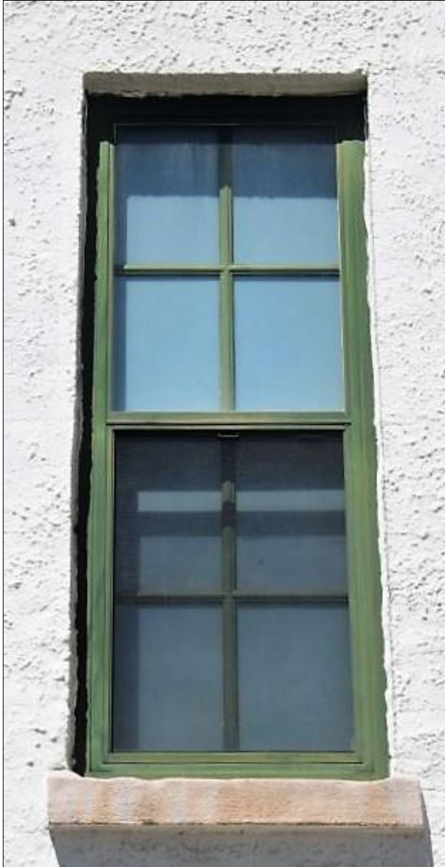
Image 2.16: Example of typical four-over-four pane window, stone plain lug sill.
