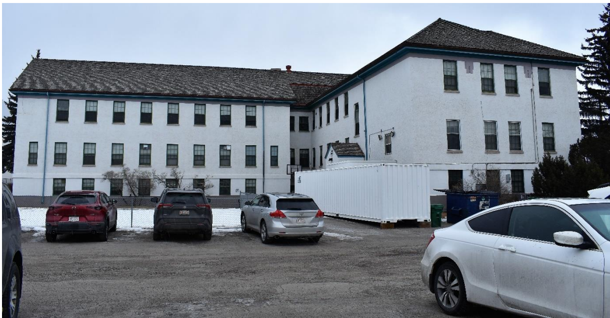
(Image 2.5: South façades, showing side portion of T-shaped floor plan)
