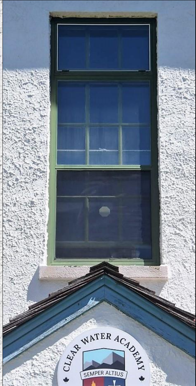
Image 2.17: Example of typical nine-over-six pane window, stone plain lug sill.
