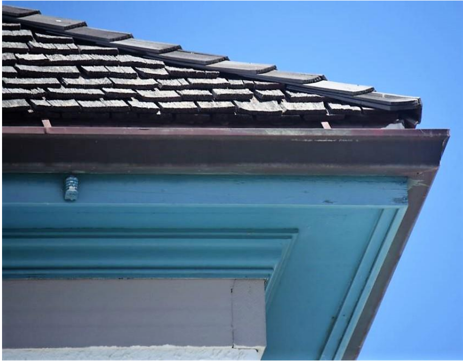
(Image 2.6: Detail of hipped roof cornice ends and cornice moulding)
