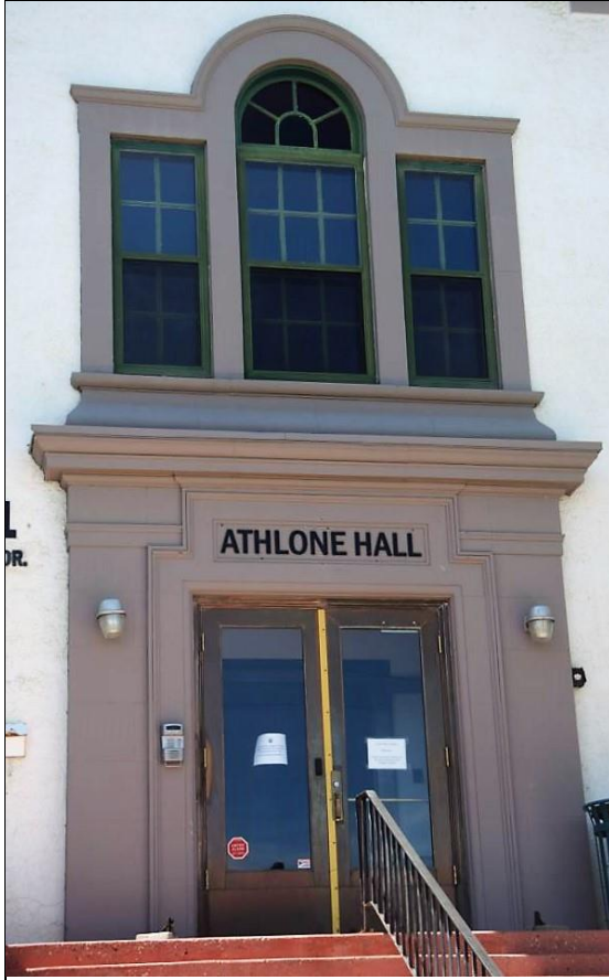
Image 2.9: Detail of Palladian window, surrounding stone pilasters.
