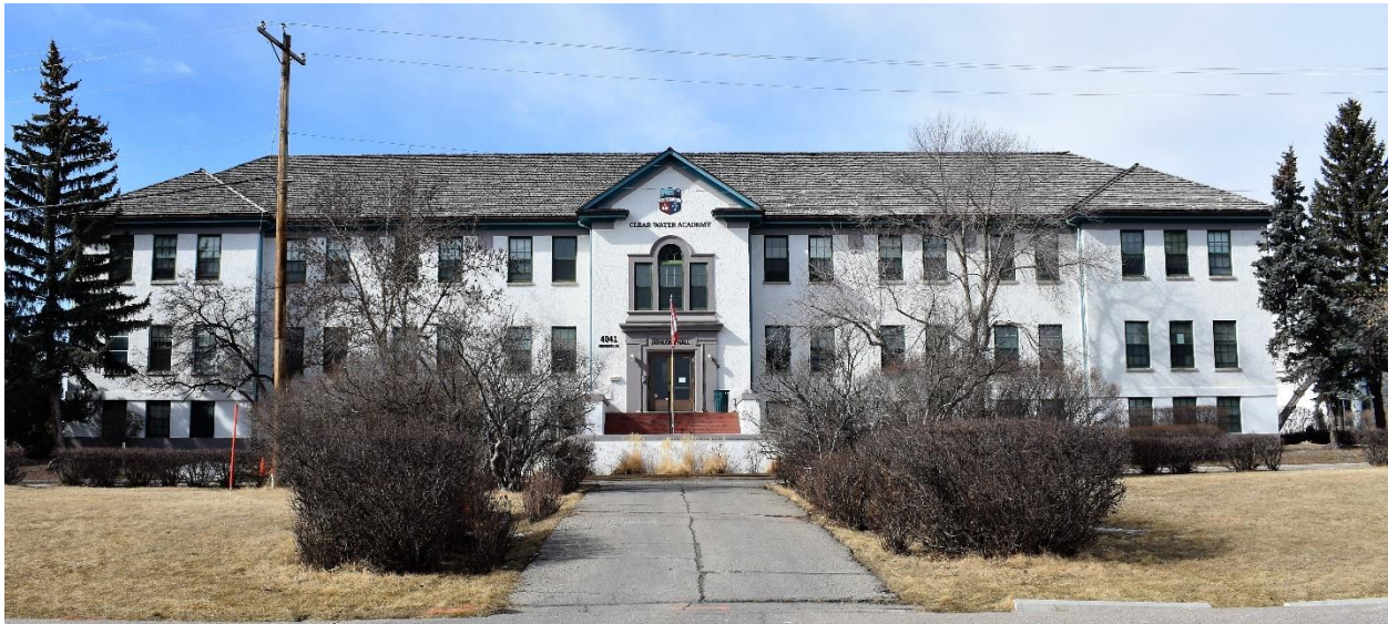
(Image 2.1: East façade with central projecting front entry pavilion, twin end pavilions)
