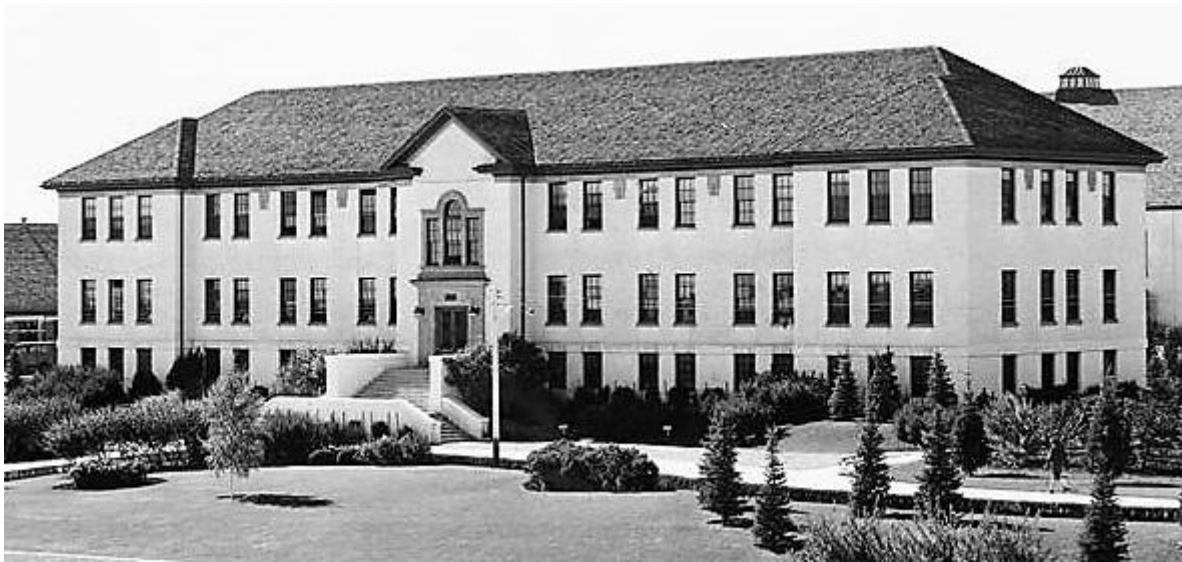
Image 2.2: East and north façade, no date, Glenbow PA-3439-9)
