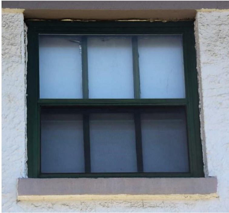
(Image 2.14: Example of typical three-over-three pane window, stone plain lug sill)
