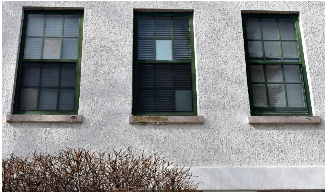
(Image 2.13: Typical fenestration, six-over-six pane windows, stone plain lug sills)
