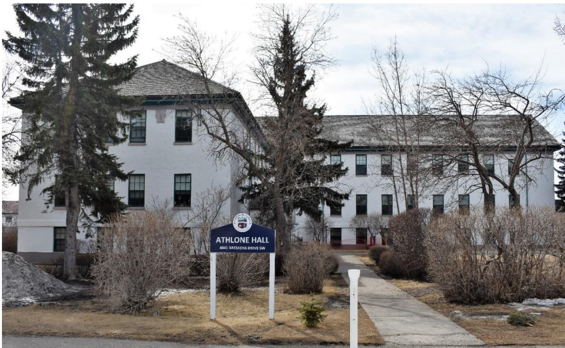
(Image 2.3: North façades, showing side portion of T-shaped floor plan)
