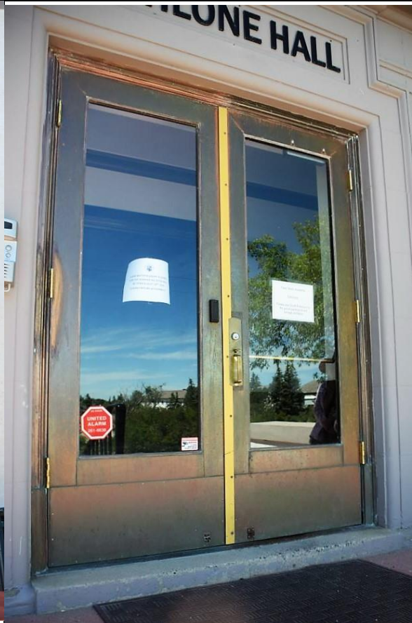
Image 2.10: Glazed brass double front entry door, metal door frame.
