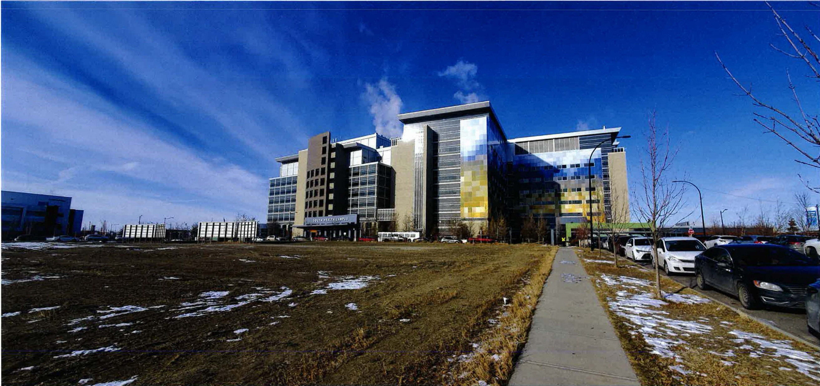
View of the South Health Campus looking
