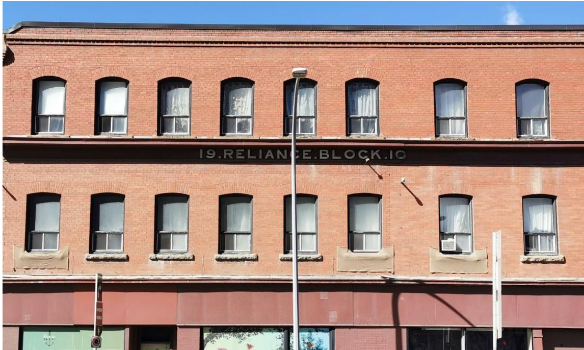
(Image 1.4: Detail of fenestration on 1909-11 building portion; segmental-arched window openings; jack arch brick headers; sandstone window sills)
