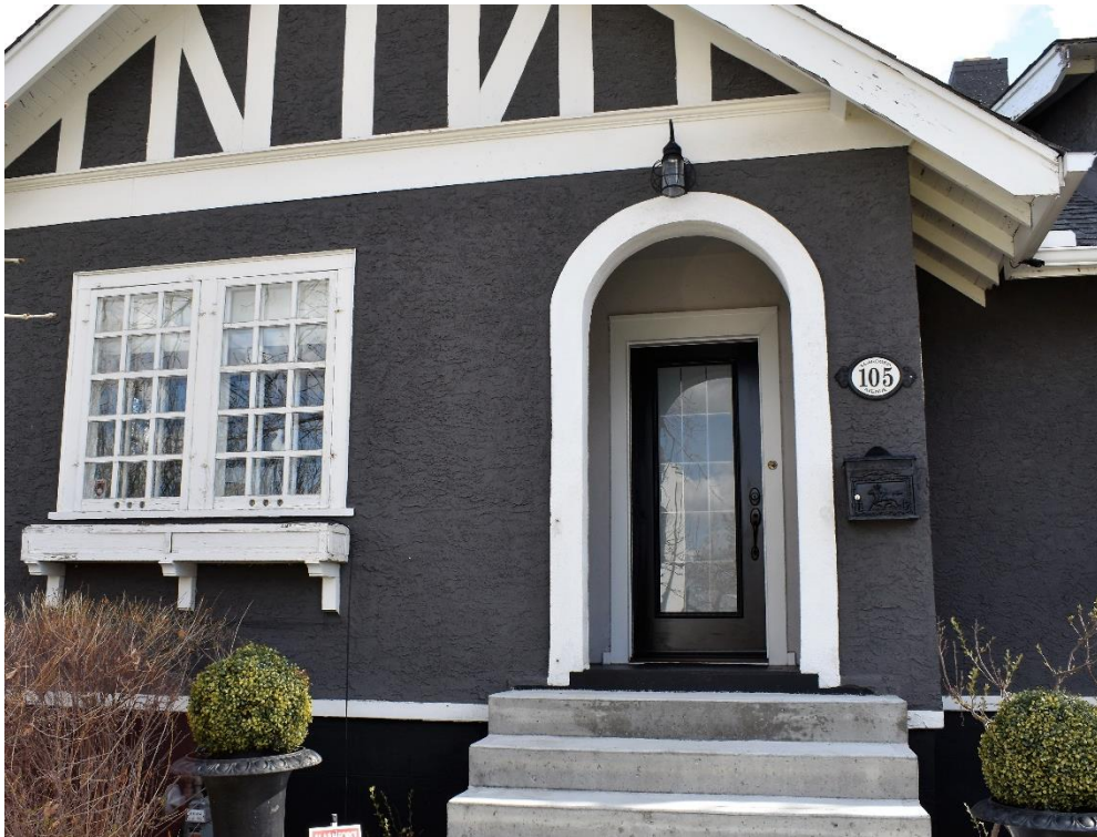
(Image 2.8: Detail of front entry recessed behind wood rounded arch offset under north gable)
