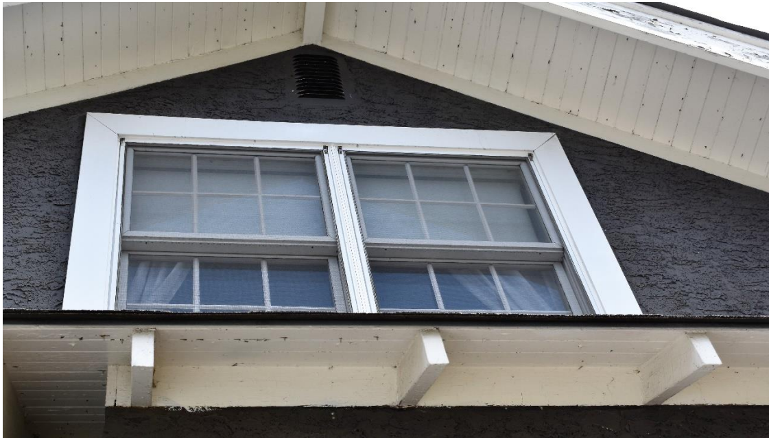
(Image 2.6: Detail of wood tongue-and-groove soffits and exposed rafter tails)
