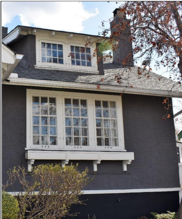
Image 2.10: Typical twinned and triple multi-pane single-hung window assemblies
