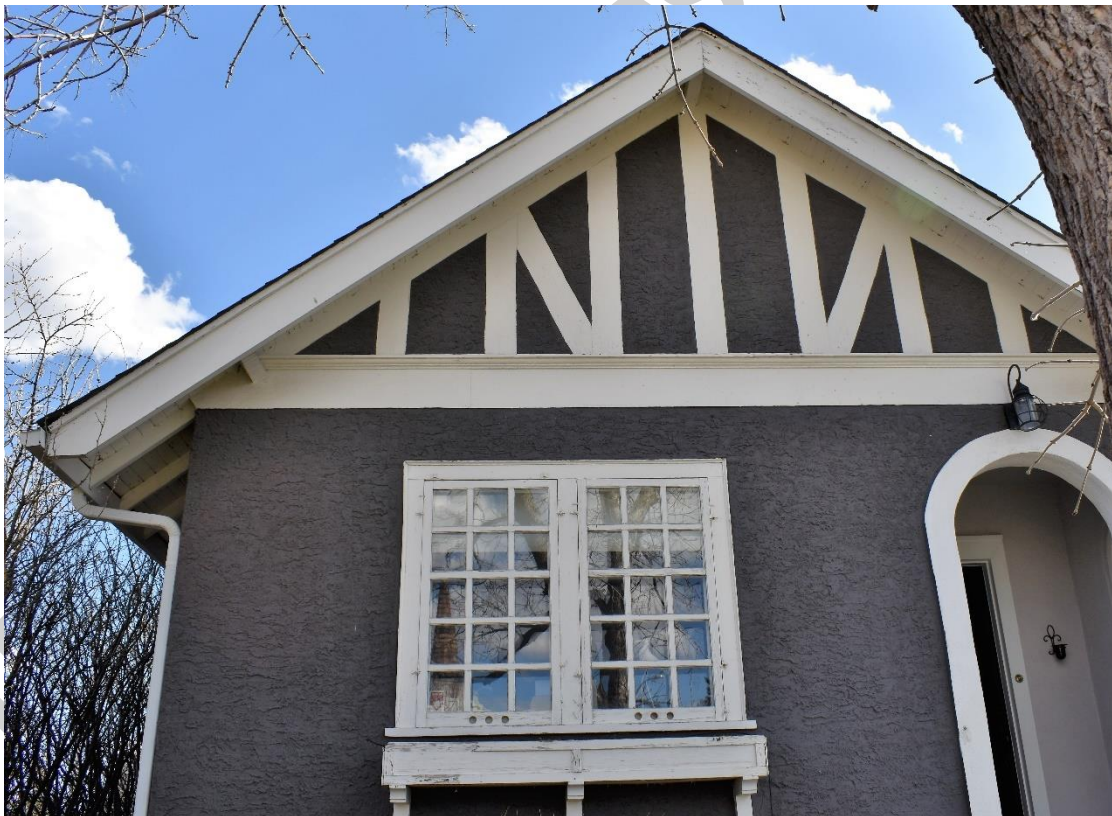
(Image 2.7: Detail of moulded wood verge and mock half-timbering on north gable)
