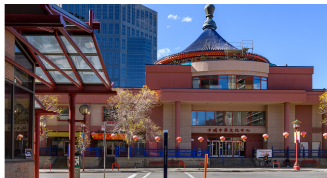
Calgary Chinese Cultural Centre, constructed in 1992
