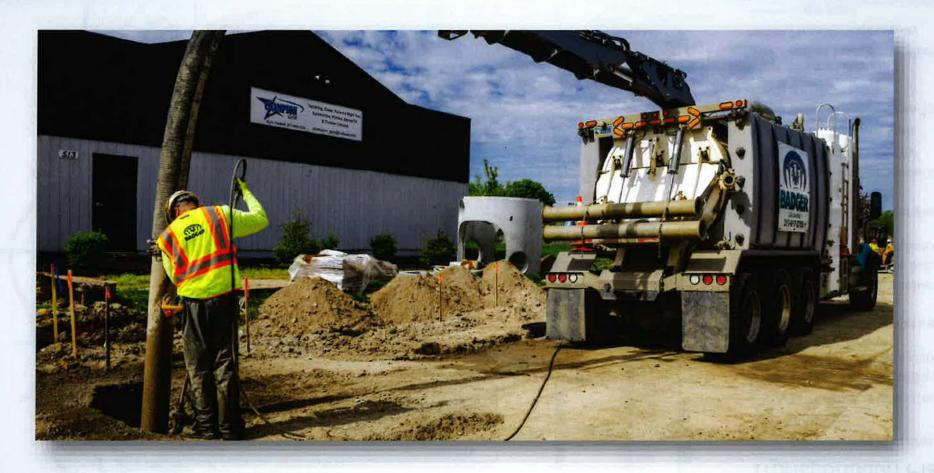
Hydrovac excavation is a precise, non-mechanical, non-destructive process that uses pressurized water and an industrial strength vacuum to simultaneously excavate and evacuate soil. As the pressurized water breaks up the soil it creates a slurry that is removed by a powerful vacuum into a debris tank.
