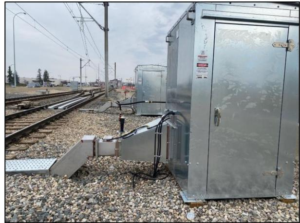
Figure 6: New switch heater with snow sensor in Whitehorn
