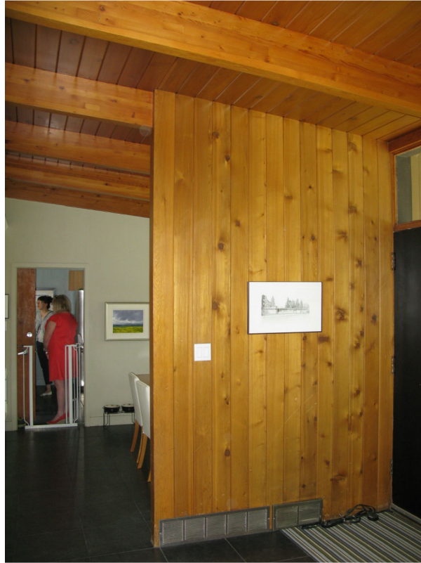
(Image 7.5: Knotty Red Cedar interior paneling and Douglas Fir glulam beams in foyer and dining room)
