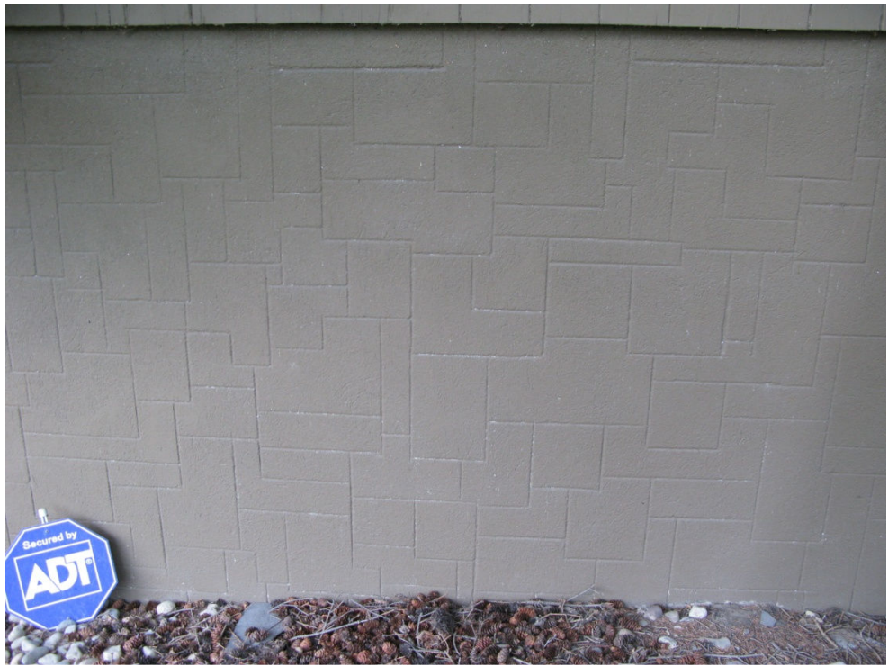
(Image 3.7: An example of the scored concrete foundation)
