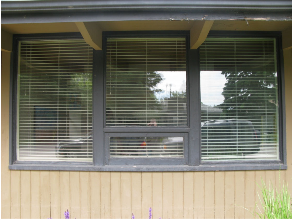
(Image 2.6: An example of the wooden-sash windows with awning opening)
