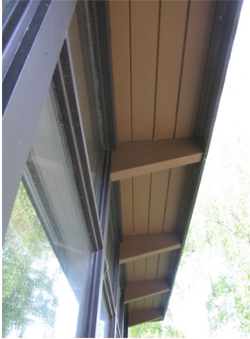
(Image 6.2: an example of the open eaves with exposed beams)
