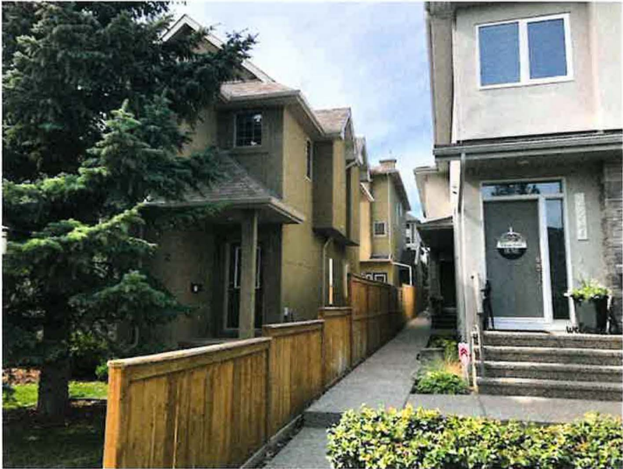
- View from the NE corner (on 29 th St SW)
