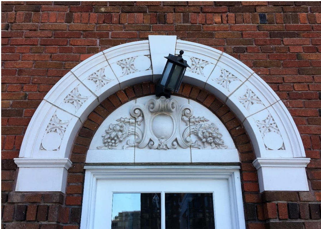
(Image 1.7: Detail of terra cotta arch, brick arch and lunette panel)
