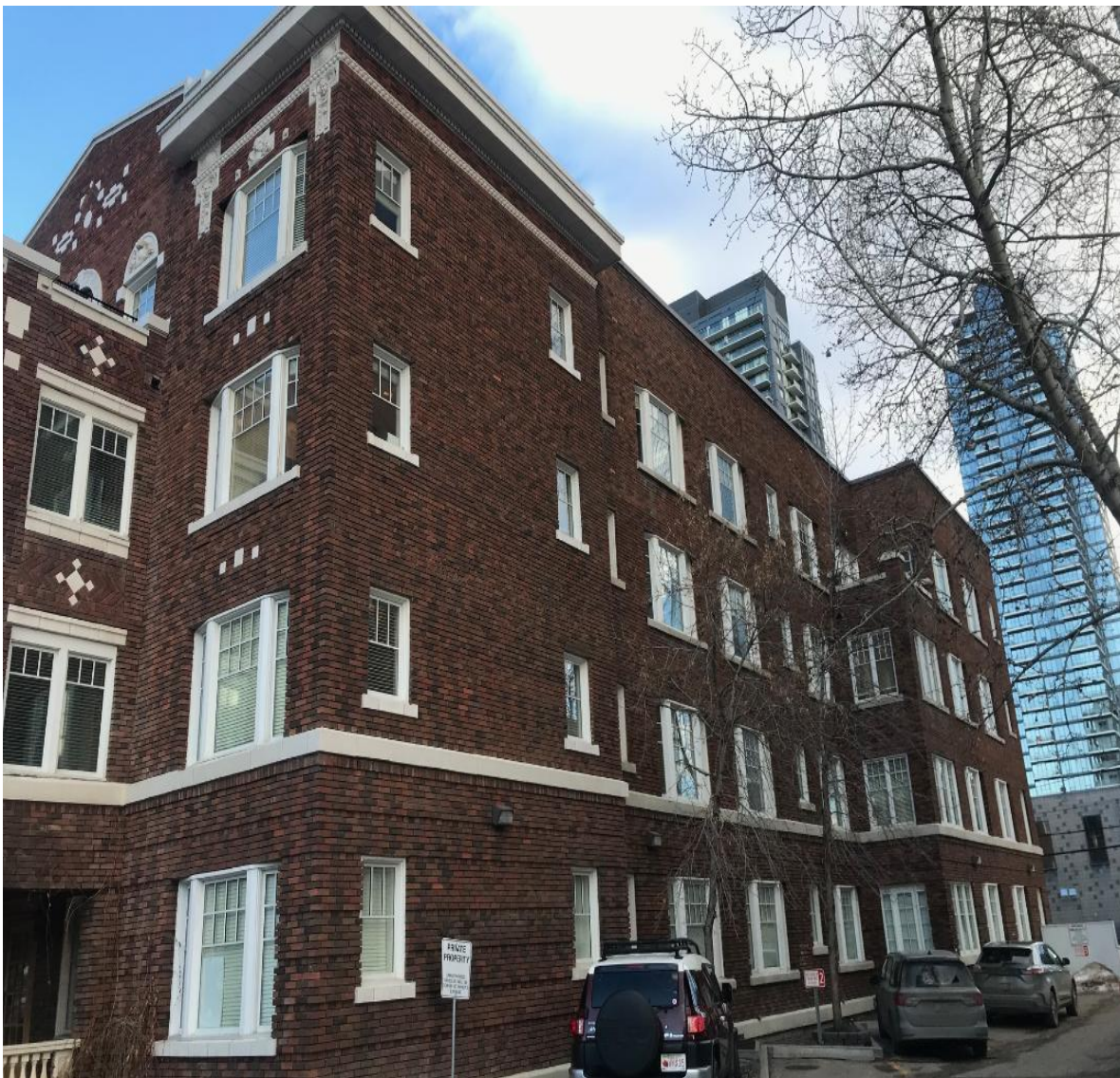
(Image 2.1: East façade looking northwest and pre-cast concrete with faux glaze band course between ground and second storeys)
