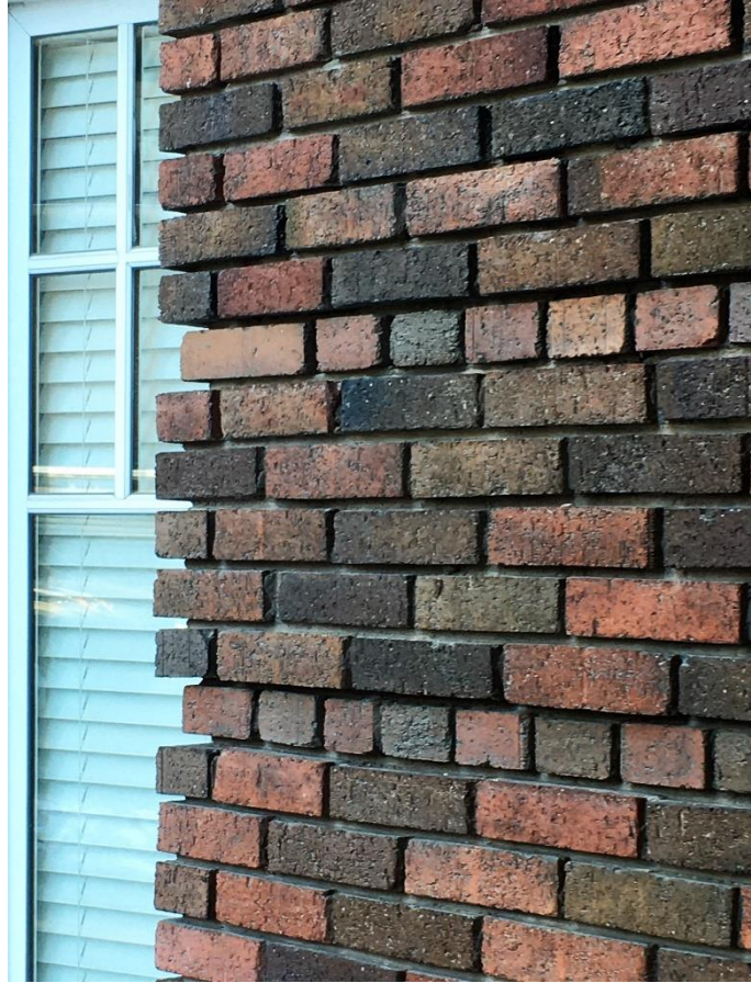
(Image 1.2: Detail of rough-textured, reddish-brown brick, recessed header rows and recessed mortar joints)
