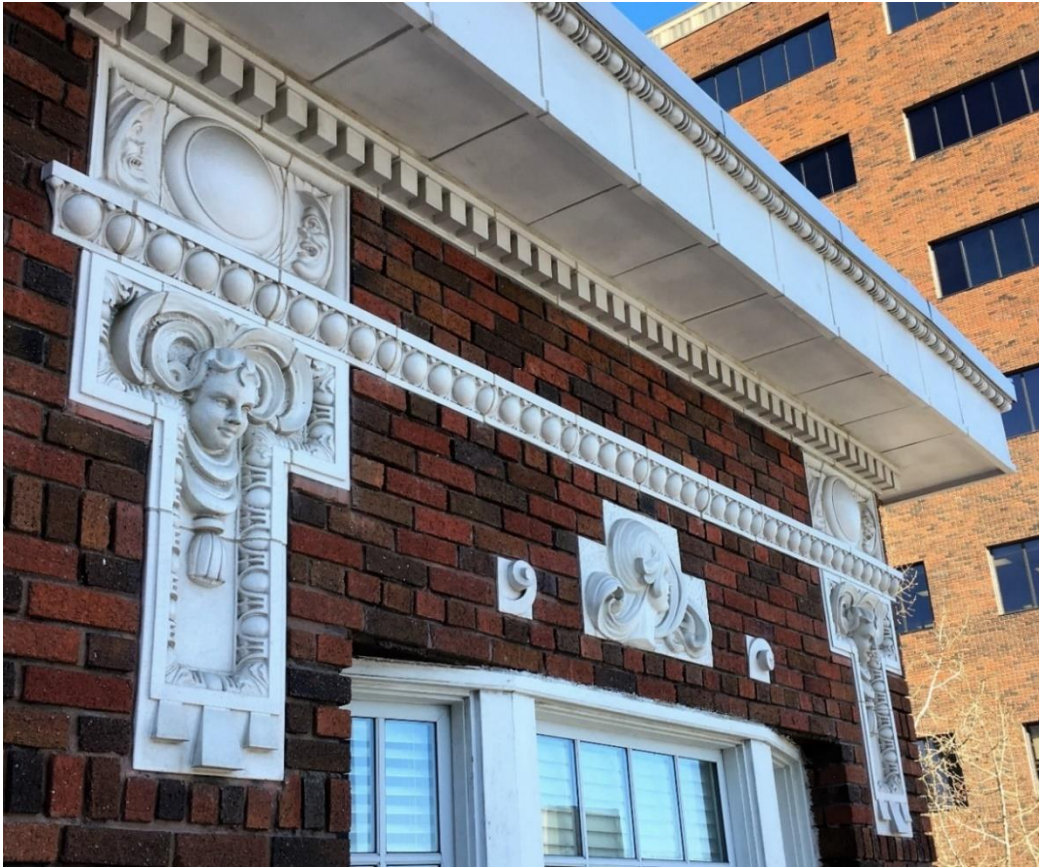
(Image 1.4: Detail of terra cotta cornice, string courses in bead-and-reel, dentil and pearl string and cartouches)
