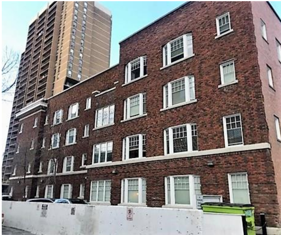
(Image 2.2: East façade looking southwest)
