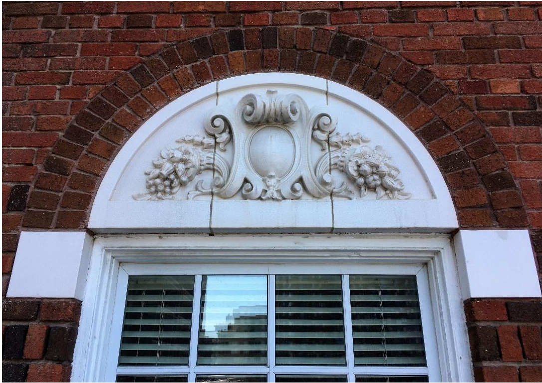
(Image 1.8: Detail of doubled brick arched header and terra cotta lunette panel)
