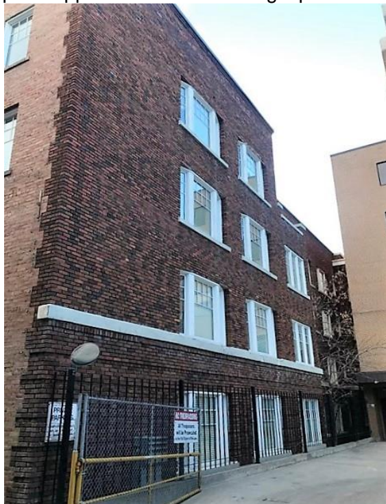
(Image 2.5: West façade at rear of building)
