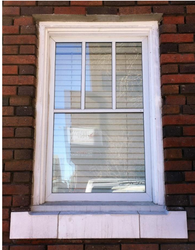
(Image 2.4: Typical multi-pane upper sashes over a single pane window profile, terra cotta sill)
