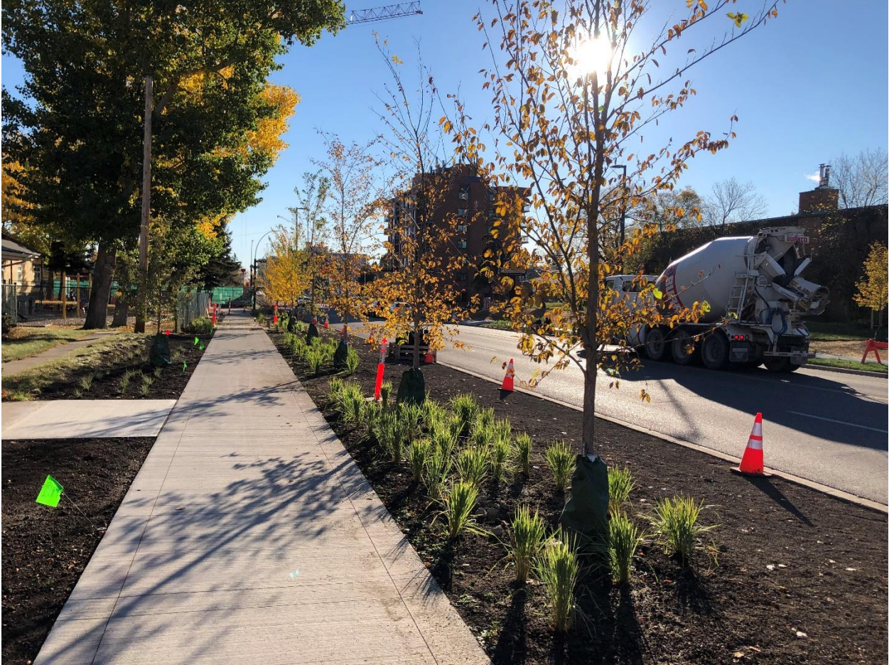
17 Avenue SW Main Street Project (37 Street to Crowchild Trail/Richmond Road interchange) – Sidewalk widening and natural buffer area allow for a more comfortable pedestrian experience.
