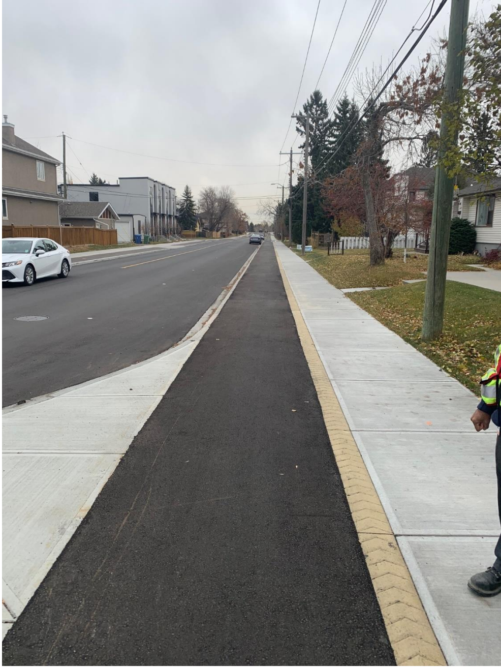
24 Avenue N.W (University of Calgary to 14 Street NW) – A raised uni-directional pathway was constructed to allow for better connectivity to the University and between communities.
