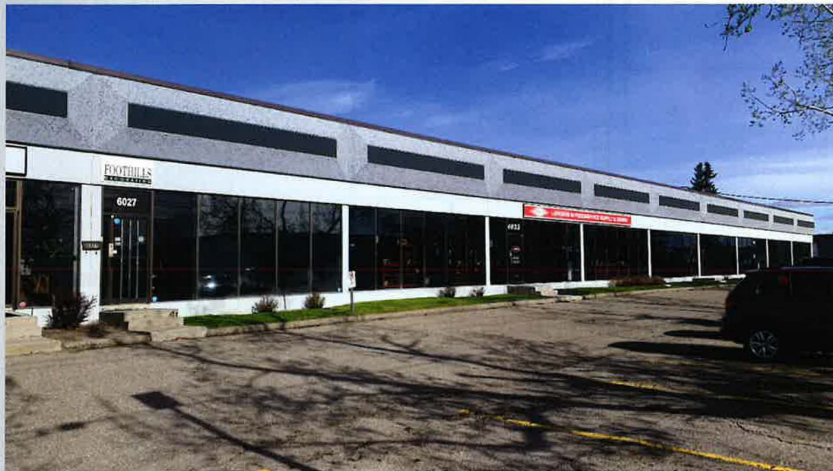
Looking South West
