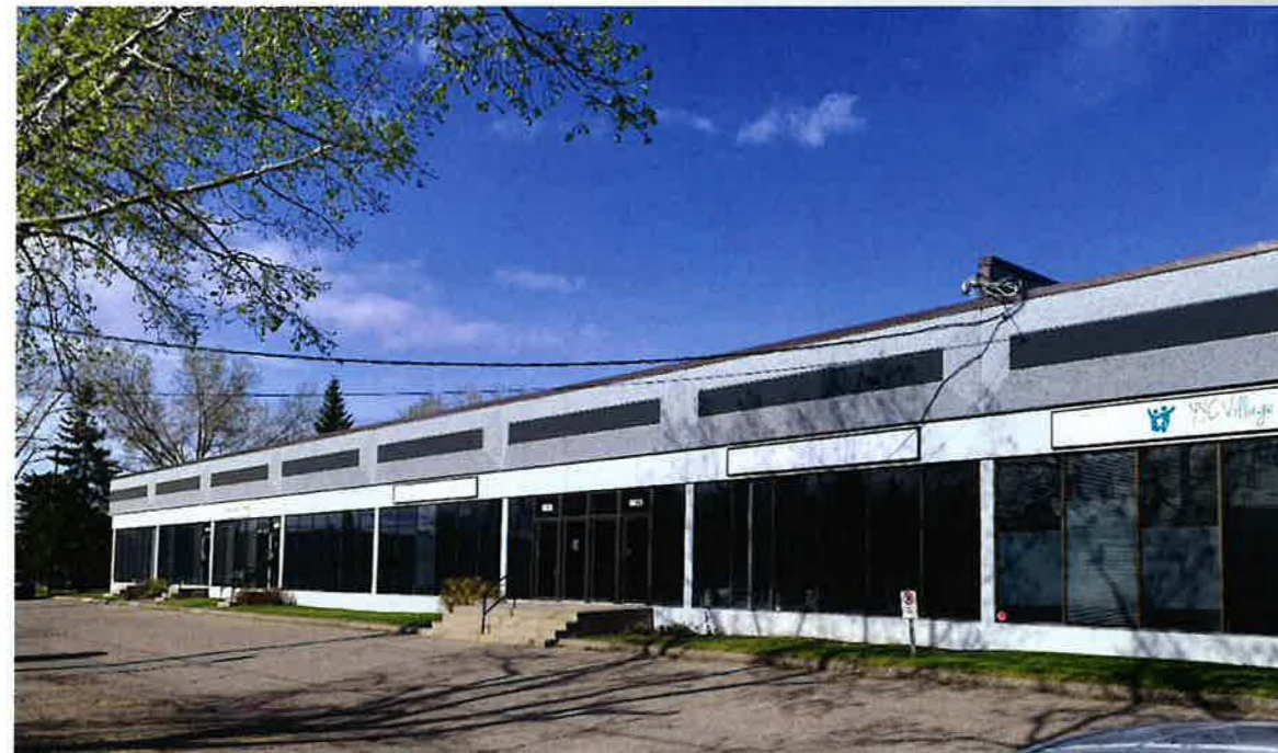
Looking North West
