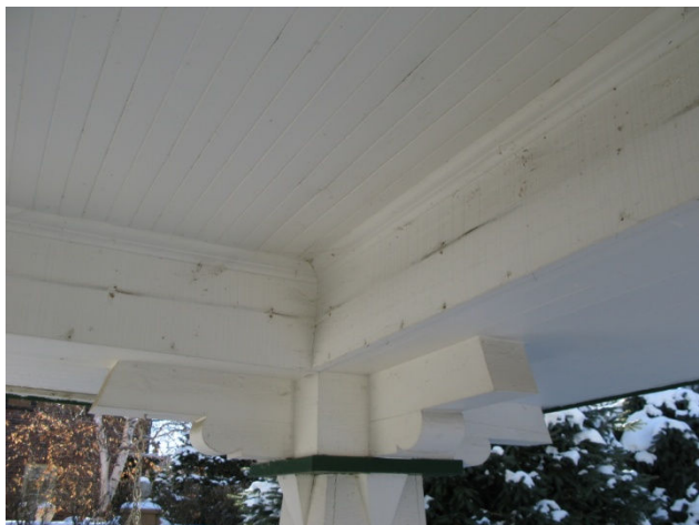
(Photo 2.5: a portion of the first storey veranda detailing showing bracketed top of column and the wooden tongue-and-groove ceiling )
