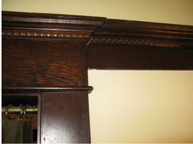
(Photo 7.8: an example of the more elaborate corniced window and casings with egg-and-dart detailing found throughout (except within the second-storey bedrooms)
