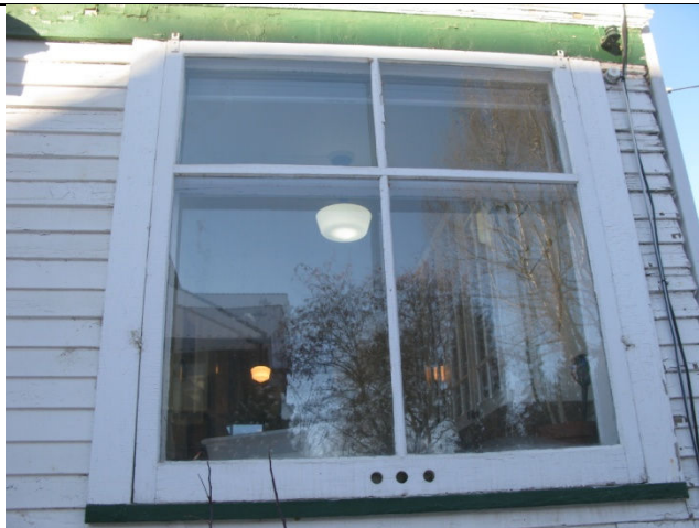
(Photo 3.4: an example of the one-over-one wooden sash windows with multi-pane storm sash)
