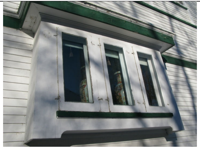
(Photo 3.5: the bay window with fixed, triple-assembly wooden sash-windows and storm sashes)
