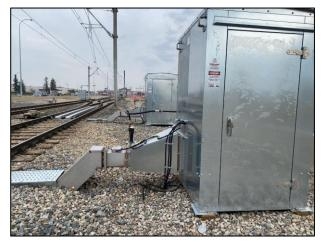
Figure 6: New switch heater with snow sensor in Whitehorn
