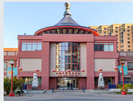
East view of the Calgary Chinese Cultural Centre from 2 Ave SW.
