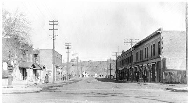
Canton Block, constructed in 1910 Glenbow Archives NC-24-52
