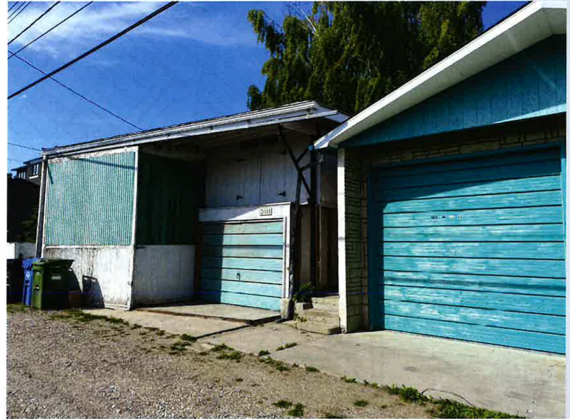
View from Rear Lane
