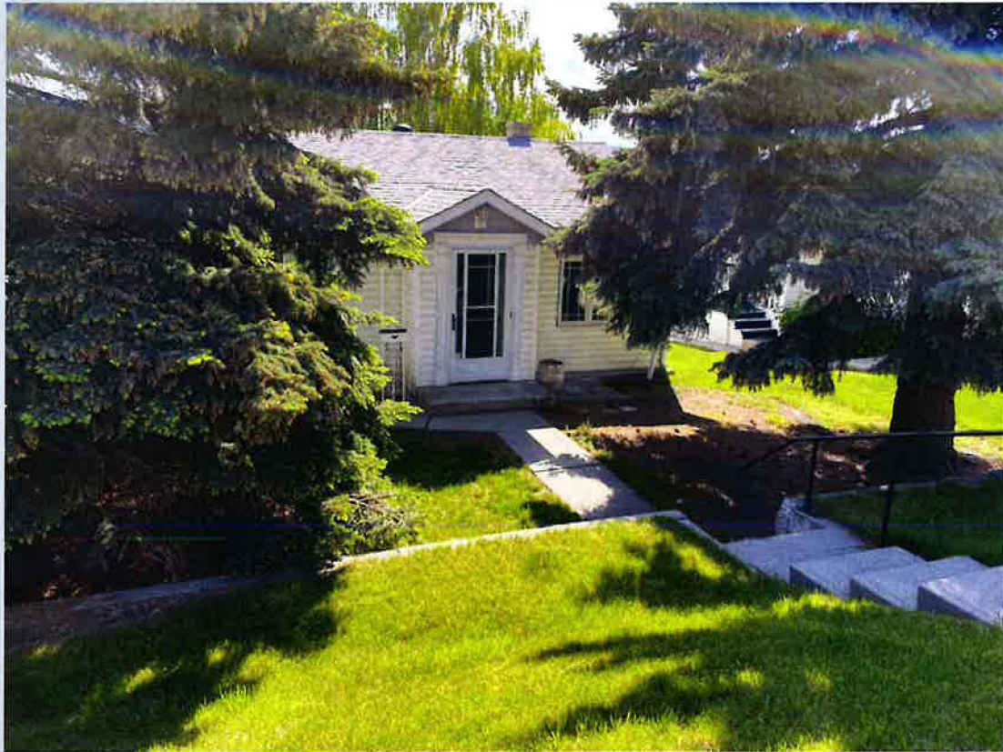
View from 22 Avenue NW
