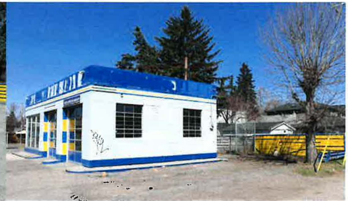
View looking northeast from southwest corner of site
