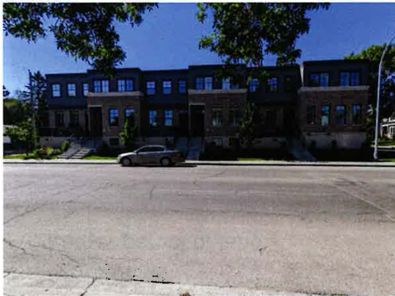
Street view from 38 Ave facing south
