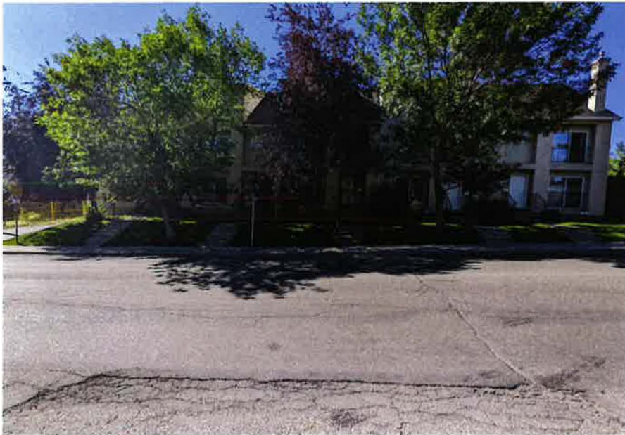
Street view from 38 Ave facing south
